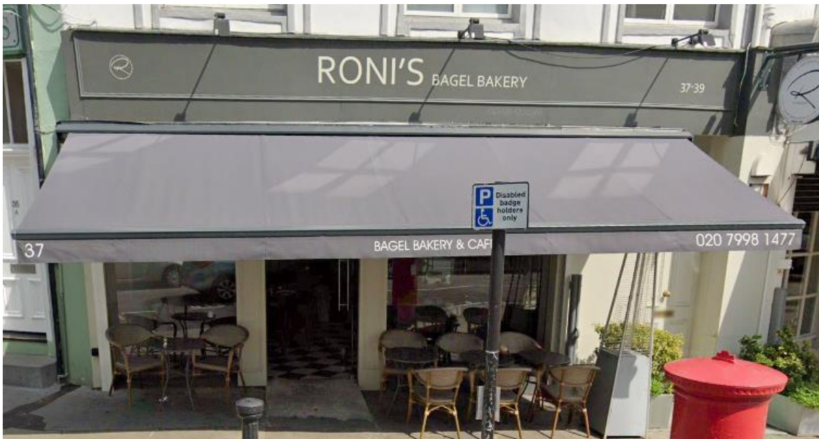
Figure 2 - Screenshot taken from google street view of the retractable awning as of July 2019
