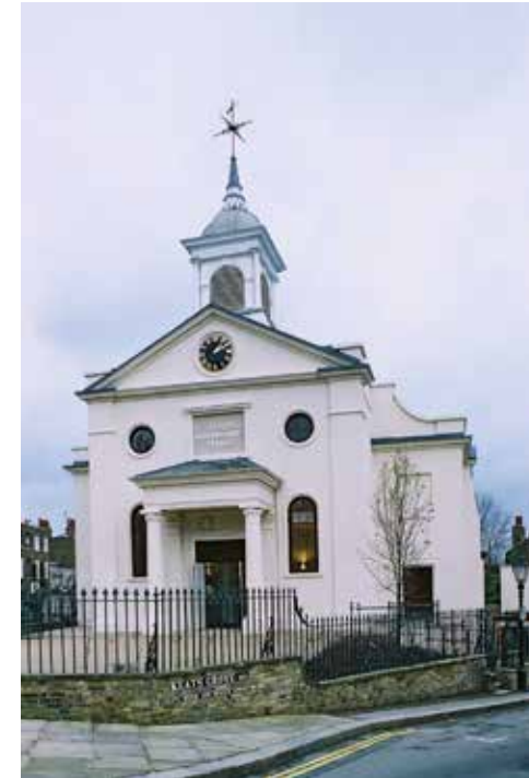
Image 4: West facade of the Church
