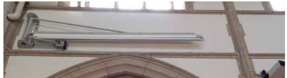
Image 8: Option 1 Precedent picture of a bespoke lever system mounted on a wall, shown in resting position
