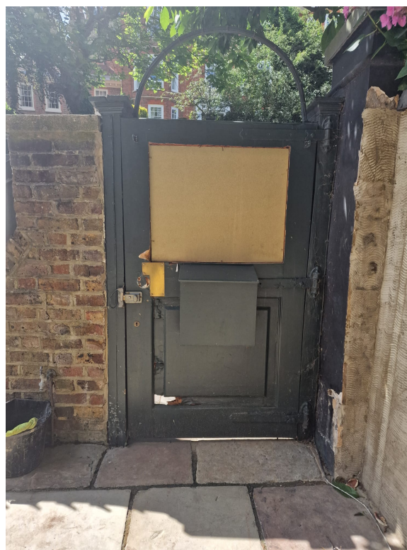
View of existing gate from rear
