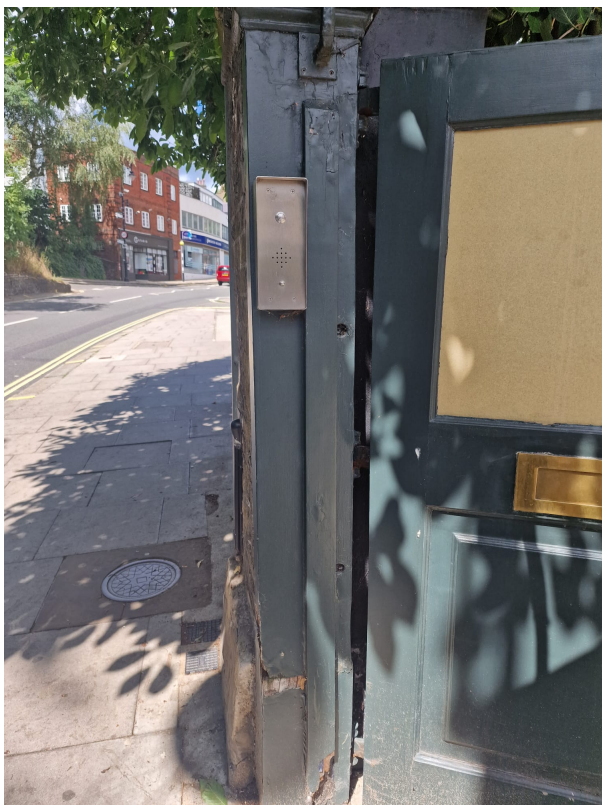
View of gate post from front
