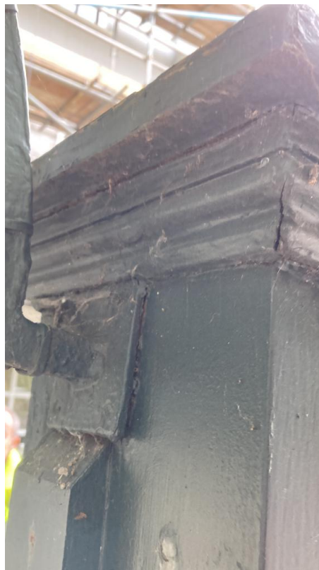
View of top of gate post
