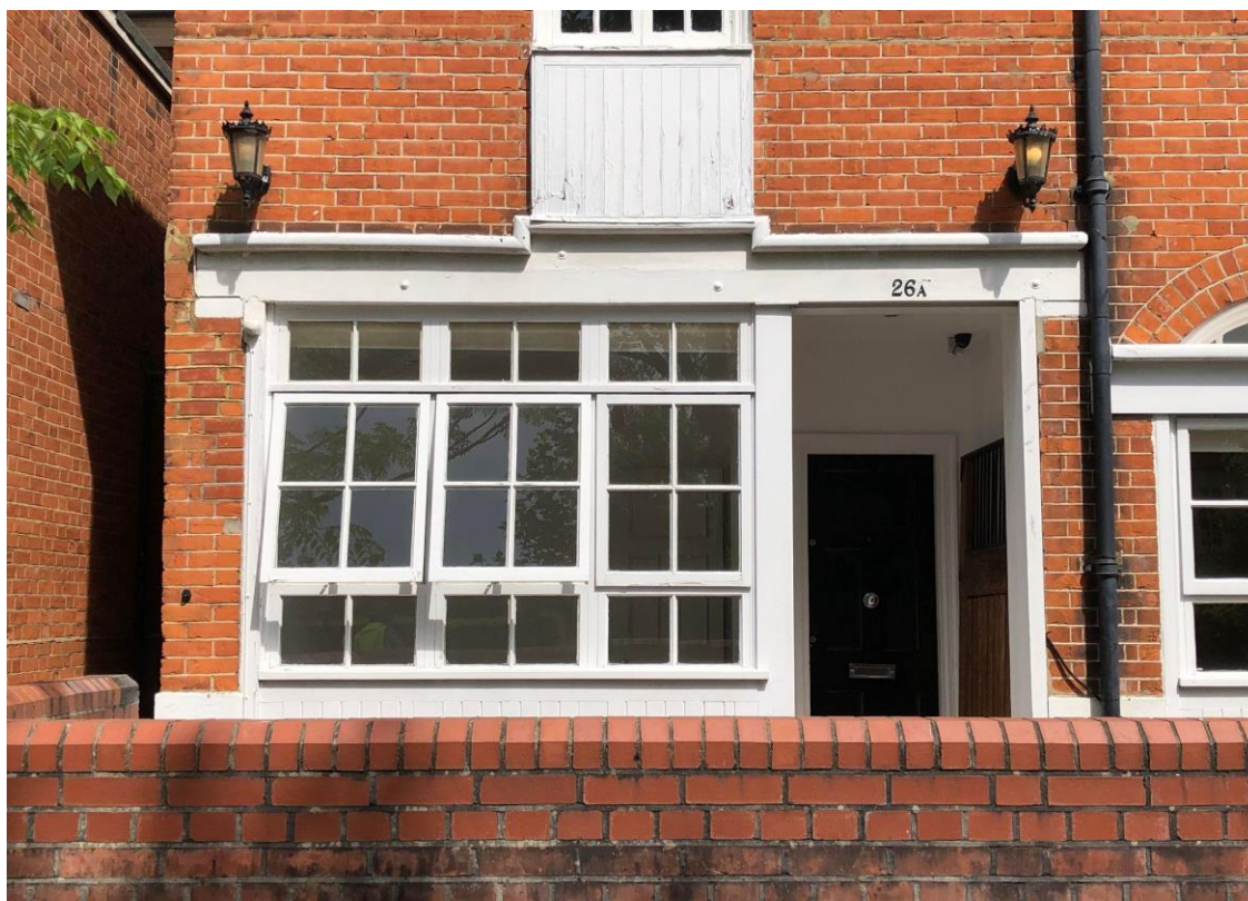
Fig 6: The former vehicle entrance originally had a pair of timber barn style doors, with the lintel being original. The existing door and windows are from the late 20 th Century and of no historic fabric value.
