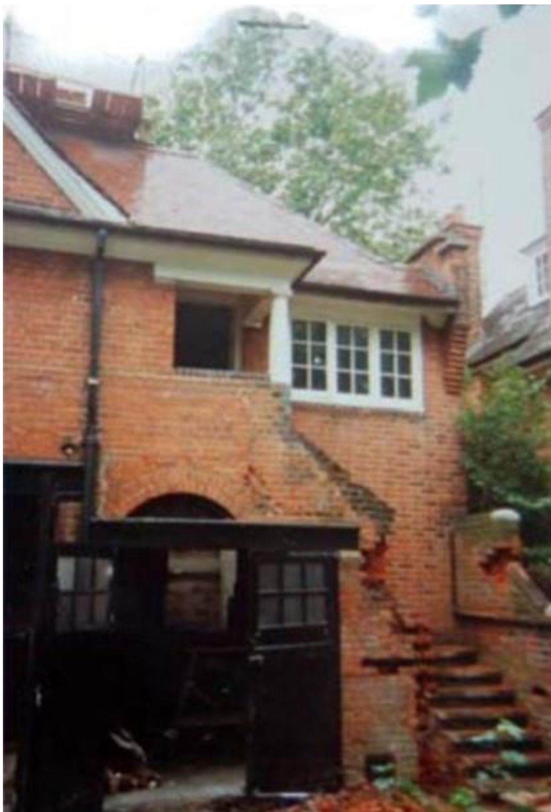
Fig 15: The photo shows the building under conversion in the 1980's with a pair of smaller garage doors in the side opening and the brickwork to the first floor staircase badly damaged and now subsequently rebuilt.
