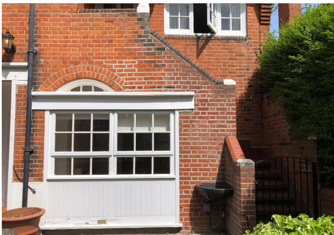
Fig 7: The historic doorway to the residential first floor will be maintained. A pair of small timber garage doors added in the 1980's will be returned to a single arched doorway, as it originally was in c.1898.
