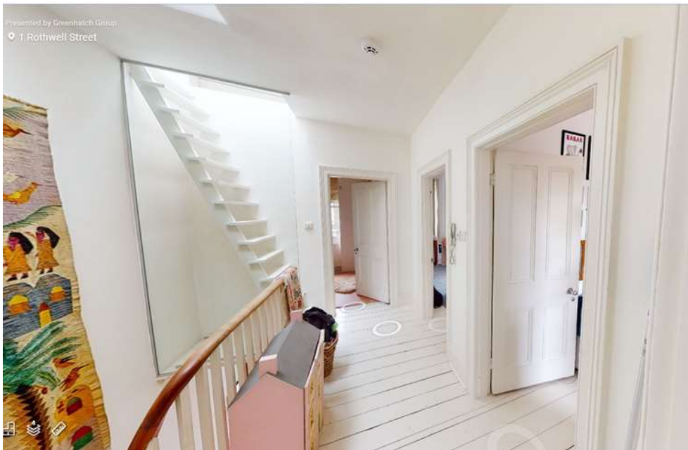
Figure 34 – view of the 2 nd floor landing. Modern glass screen replaces section of the balustrade.
