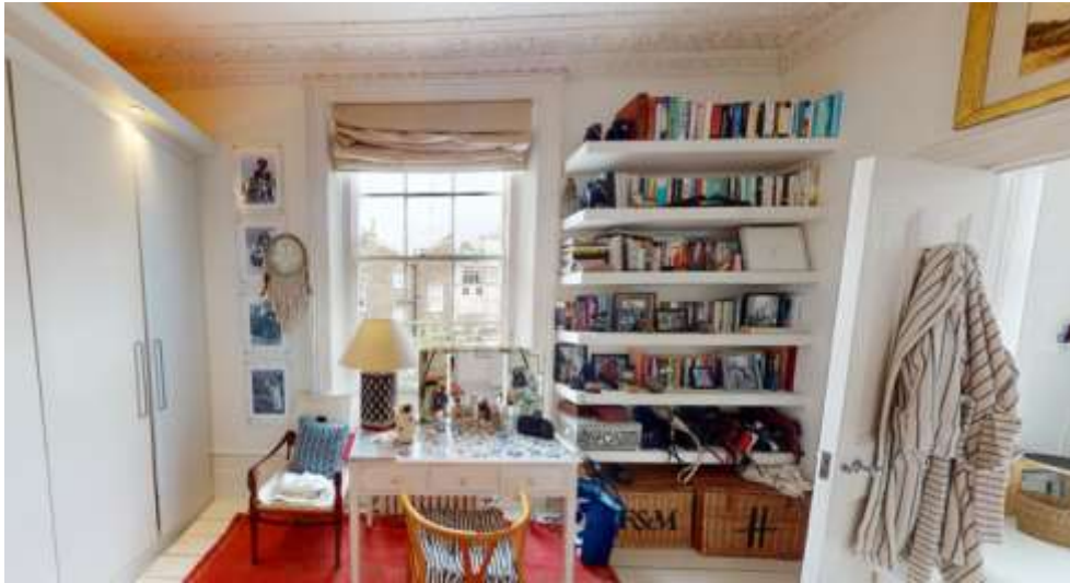
Figure 30 - This view shows 6-o-6 early timber sash window with timber architrave; Floorboards (possibly early ); elaborate cornice- same as in the front room.
