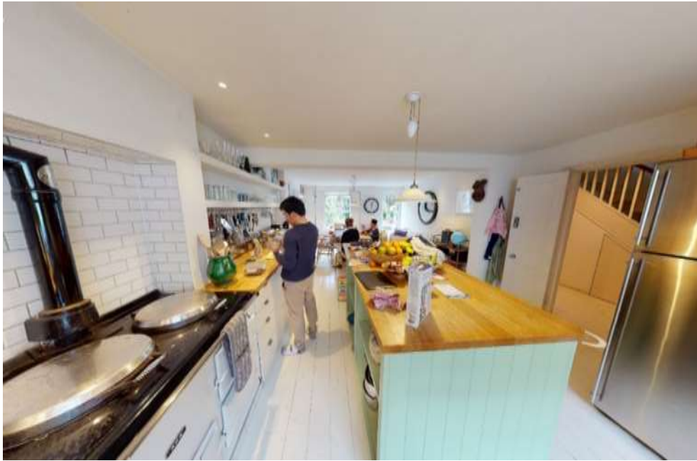
Figure 15 – View of the kitchen area. The wall between front and rear room removed with downstand beam and small nib retained. The chimney breast retained. No original fireplace/stove remains. No cornices.
