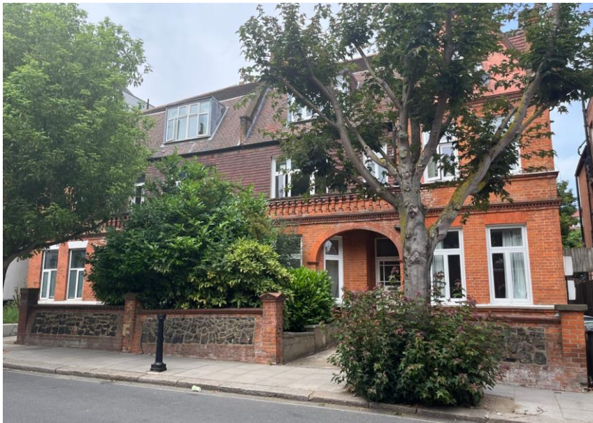
Photograph 2 Front Elevation with No.3
