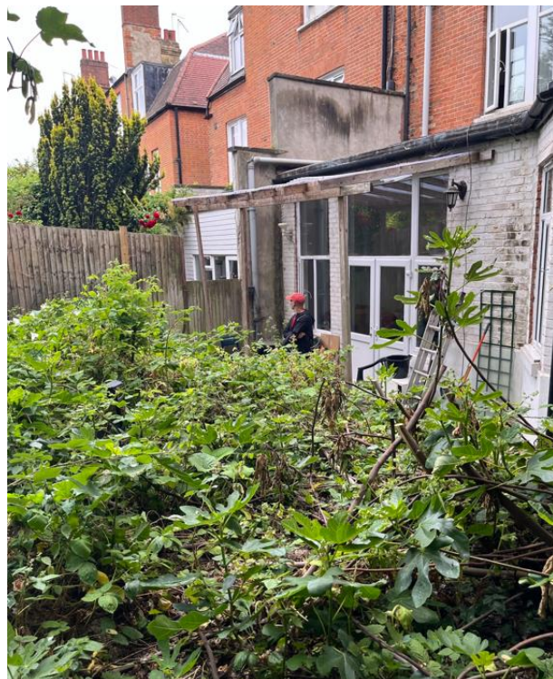
Photograph 4 Existing Rear Extension
