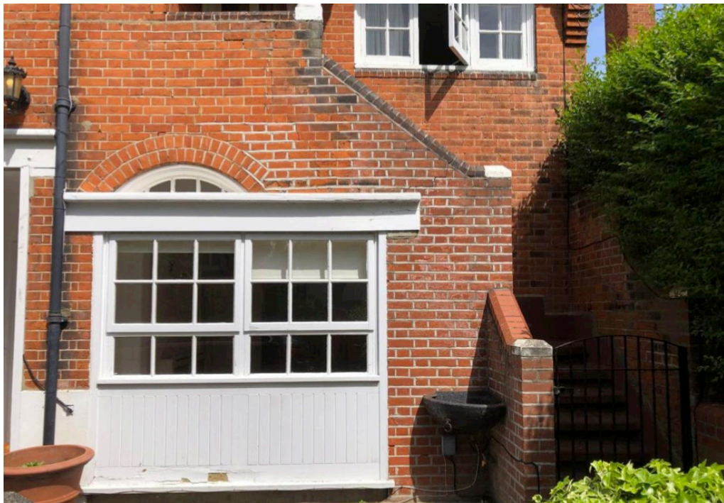
Figure 7: The historic doorway to the residential first floor will be maintained in the proposed development. A pair of small timber garage doors added in the 1980's will be returned to a single arched opening, as it originally was in c.1898.
