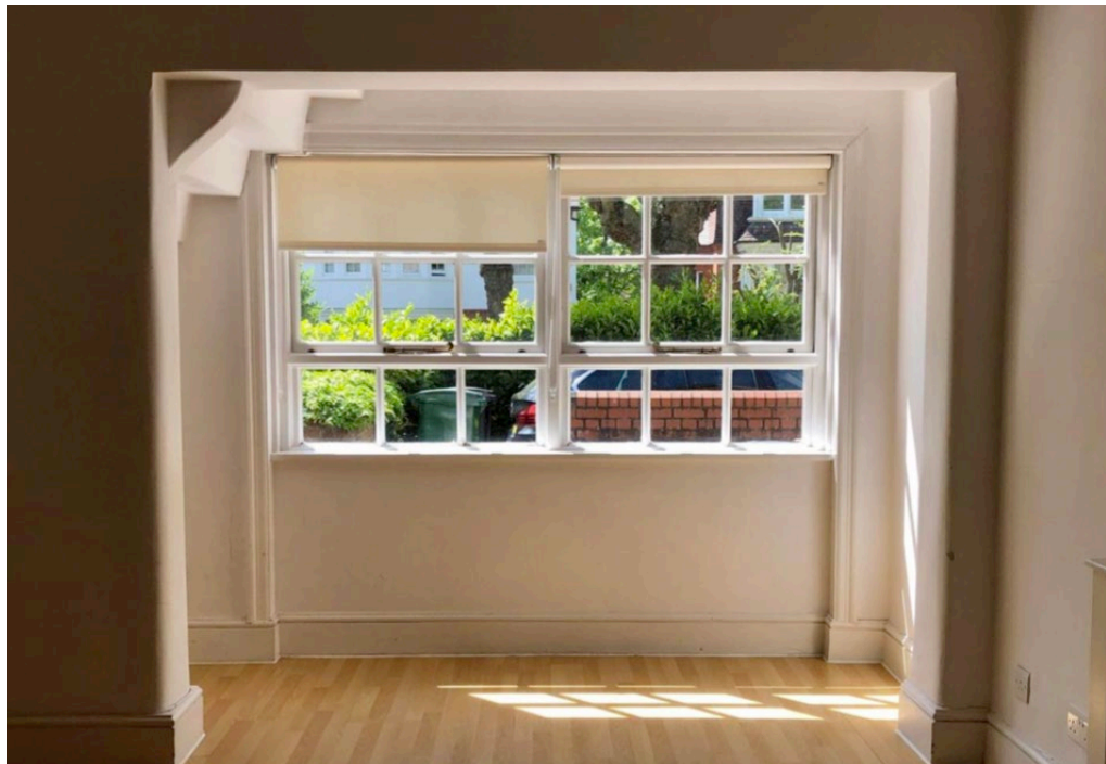
Figure 13: The existing front window does not contain any historic fabric and dates from the late 20 th Century, when the building was converted to a dwelling. Many of the internal features date from this conversion.
