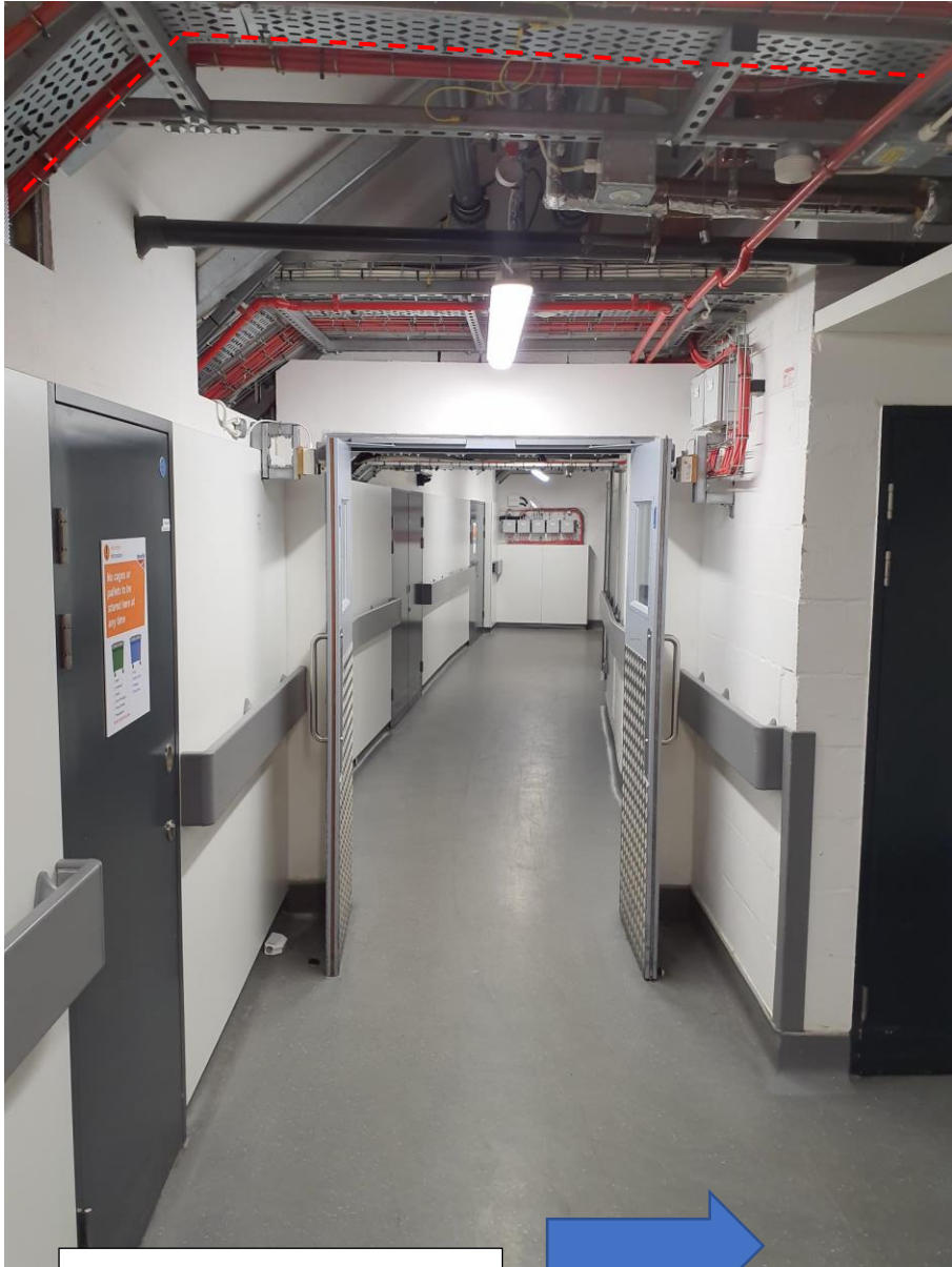
DOORS TO ACCESS MEZZ FLOOR+1 NODE 6 ROOM 123/D1N
