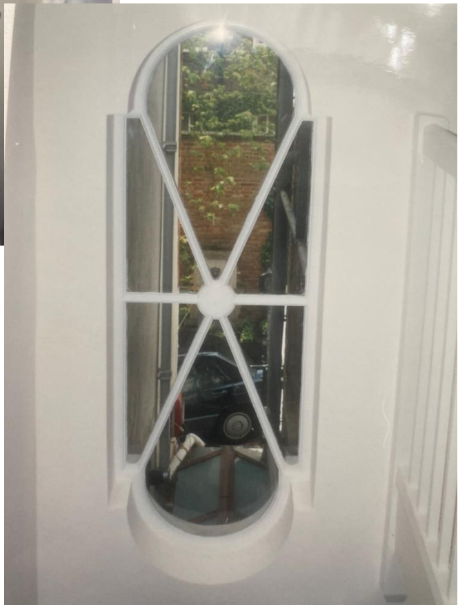
Replacement landing window.
