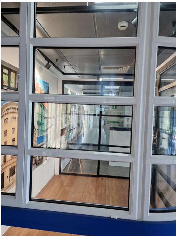
Figure 9 – picture of transom-style fixed glazing bars
