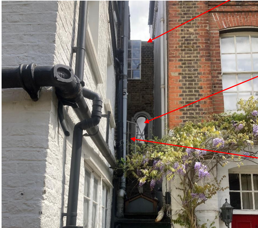
Figure 1 – Bathroom Light well
