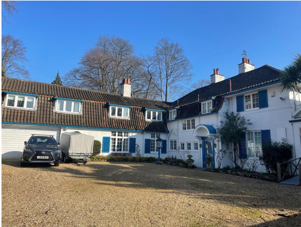
Above: Existing 'Croftway House'
