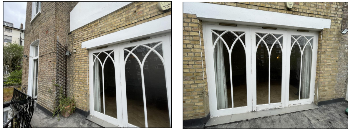
Images of Existing Rear Doors
