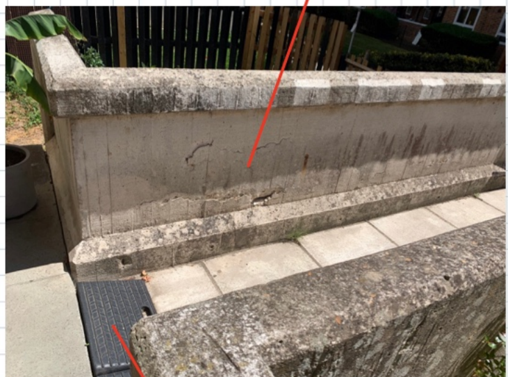
Showing spalled concrete
