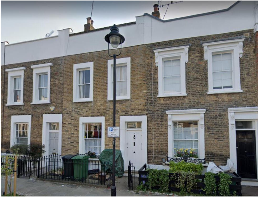
Figure 3: Front elevation as viewed from Alma St of the application site (identified with white front door).
