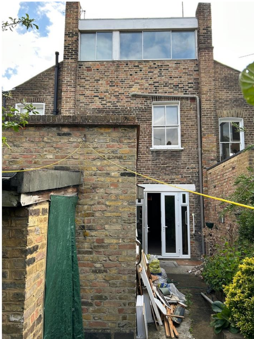
Figure 4: Rear elevation of application site.
