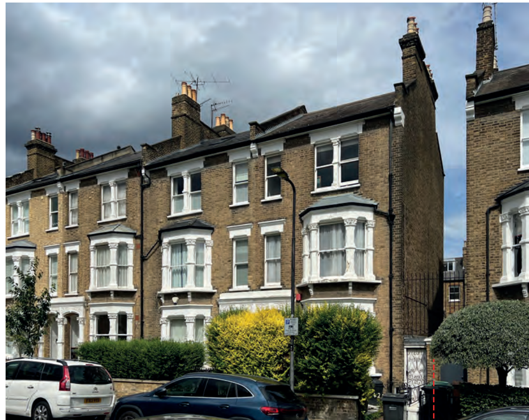
Photographs of front elevation and neighbouring properties
