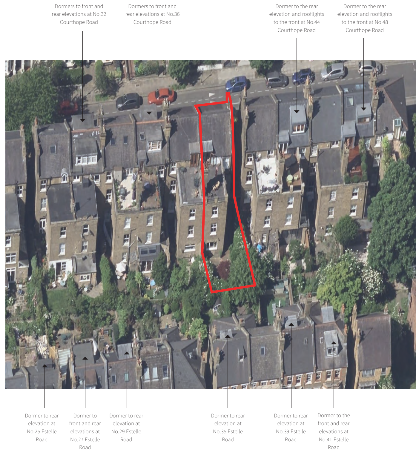
Birds-eye view of the property viewed from the east showing rear elevation and garden.
