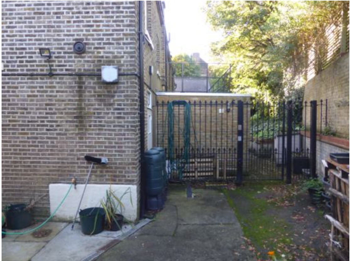
Fig.3 West range rear ground floor elevation.
