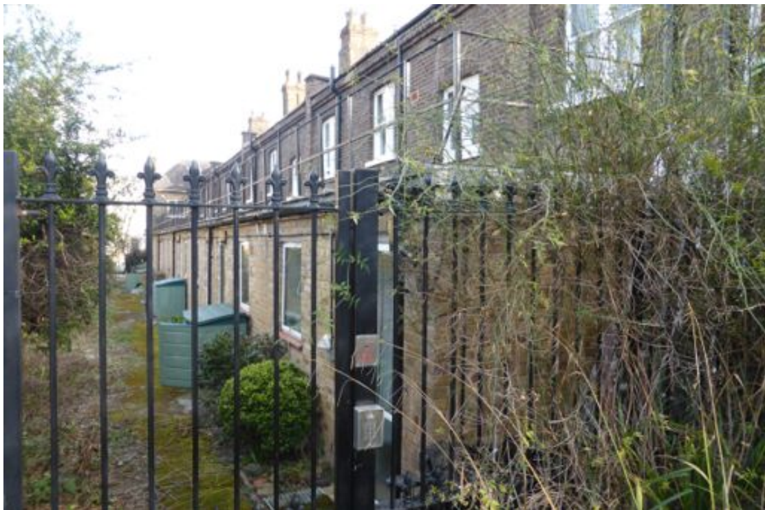
Fig.2 North range rear ground floor elevation.
