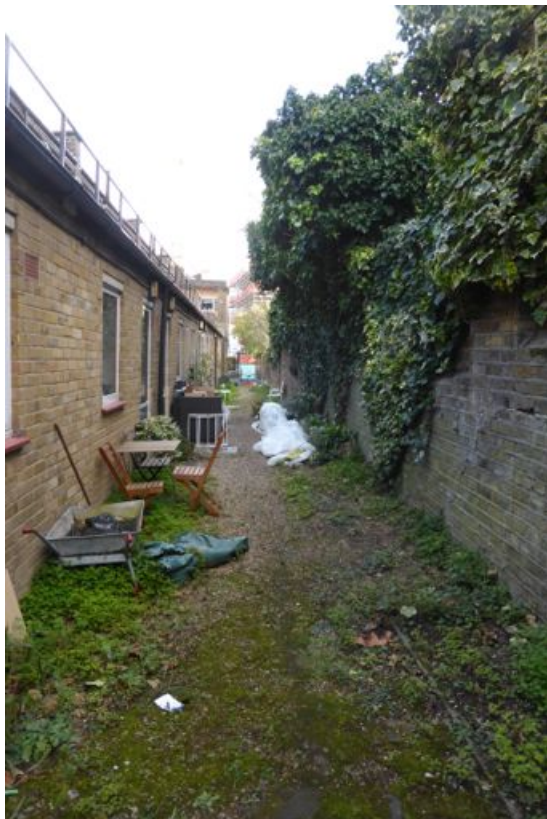
Fig.4 South range rear ground floor elevation.
