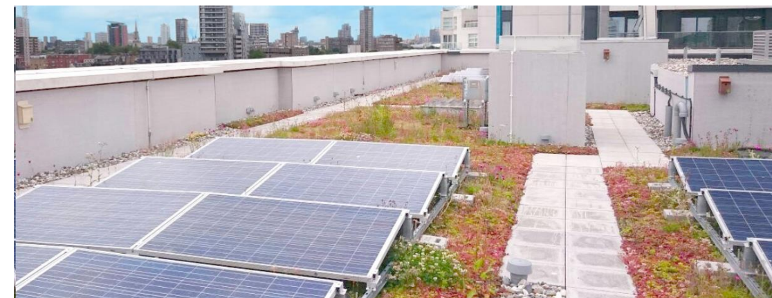
Figure 7 Van De Valk PV Green Roof PV Racking System.
