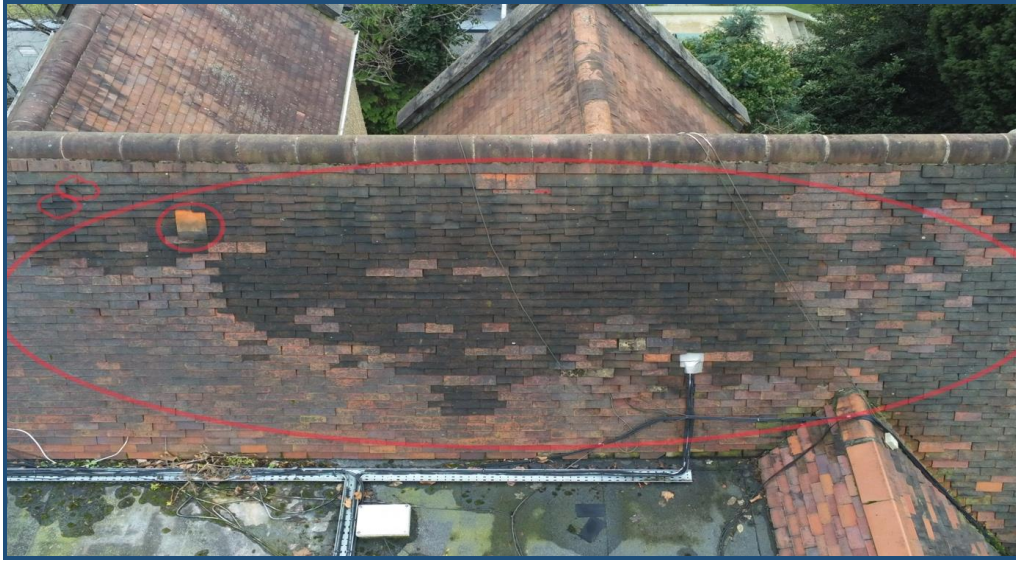
Photo No.12 - note localised past patch repairs to roof coverings.
