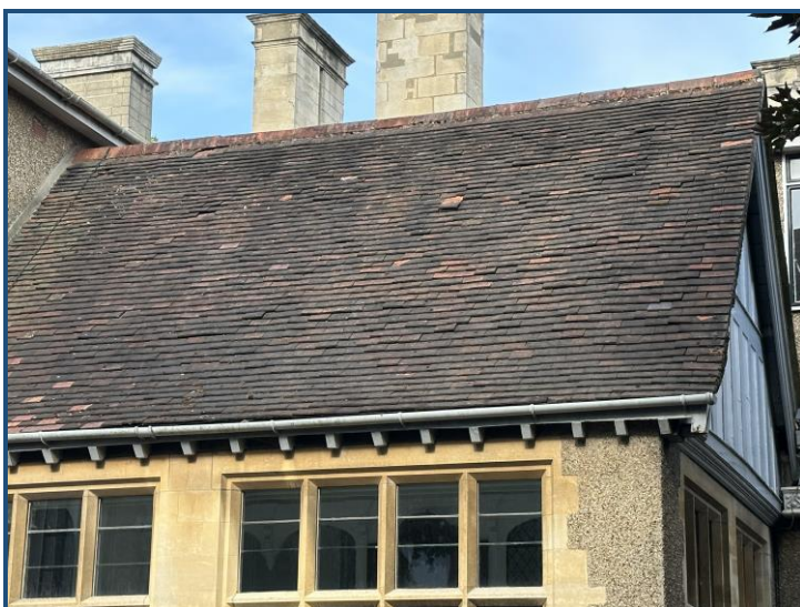
Photo No.7 - view of tiled roof coverings. Note significant slipped and lifting tiles.
