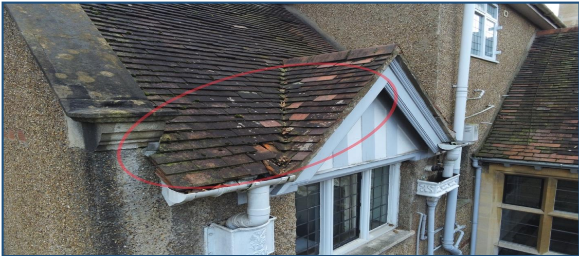
Photo No.11 - Note localised replaced tiles and other adjacent slipped tiles.
