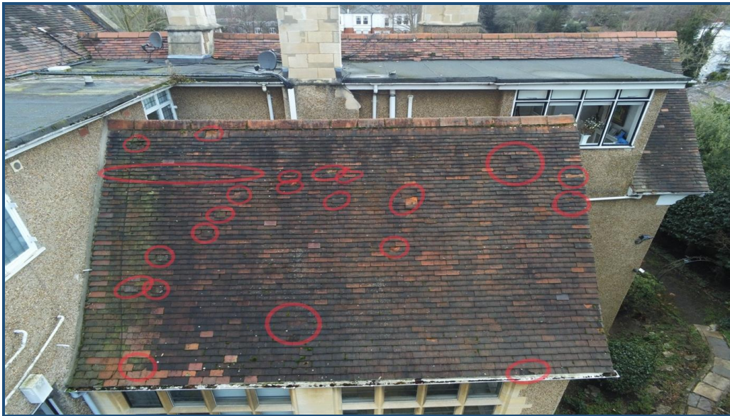
Photo No.13 - Note slipped, broken and laminated tiles highlighted in red.
