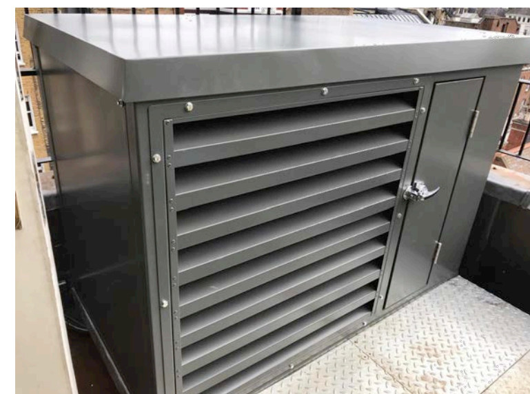
ACOUSTIC LOUVRED ENCLOSURE POWDER COATED ALUMINIUM, FLAT PANELS & LOUVRES
