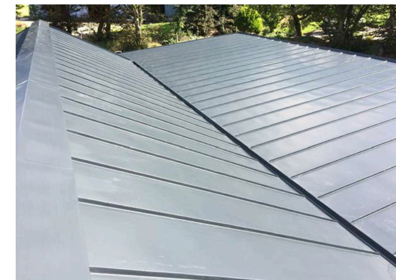
NATURAL ZINC STANDING SEAM ROOF
