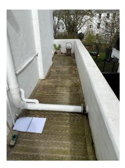
This is more of a safety issue than anything else – the soil pipe is a trip hazard and the current parapet is too low to prevent falling. In fact the entire area is dangerous without a higher form of barrier. The railings are the least visually offensive means of enclosure.
