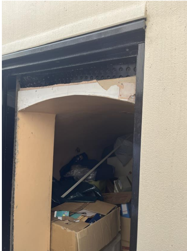
Photograph 24: Basement vaults which has had a membrane installed and have been lined below
