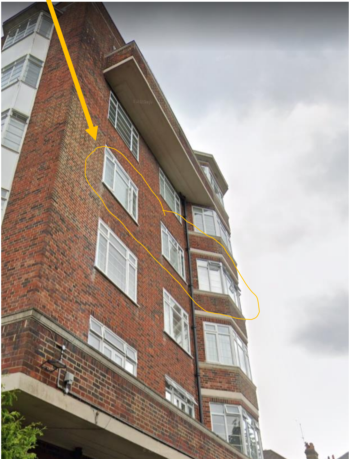
View 1 – south-west elevation showing 5 windows to be replaced
