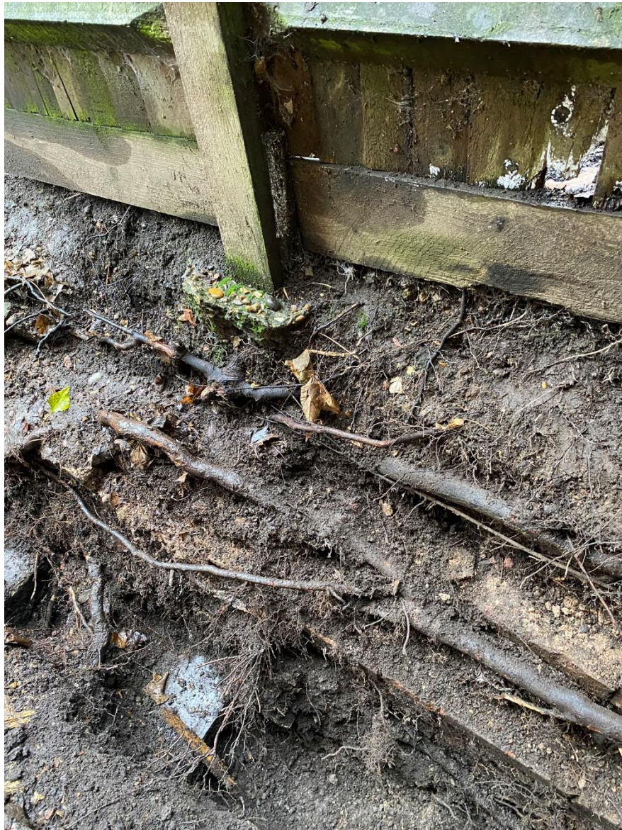
Fig.5; Trench excavations showing roots running parallel to the boundary above the capping layer. Fine, hair-like feeder roots have grown within this shallow soil but are not present within the soil in great numbers.
