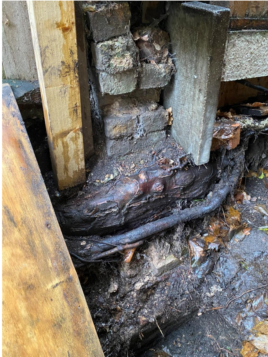
Fig.4; Root bole of T1 shown approx. 200mm below ground level, with gravel board of boundary fence as evidence of site levels. The structural root of T1 can be seen wrapping around a brick pillar.
