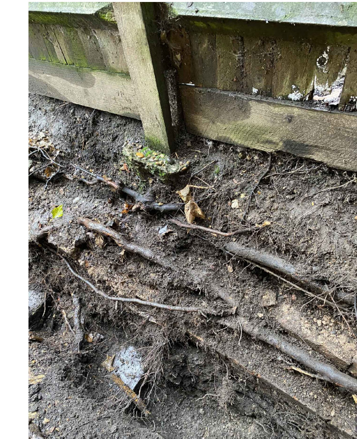
Figure 1: Trial pit excavations along the boundary with the car park revealed that root growth of T1 and TG2 has proliferated along the top of a historic boundary wall. The trial pit revealed roots have not grown beyond the boundary wall and trespass is limited to fine, hair-like roots within the soil on top of the sunken structure, therefore structures inside of this boundary would have no harmful effect on tree roots.
