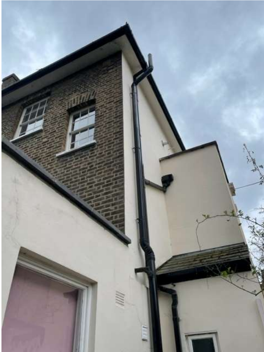
Side (flank elevation) at rear elevation return
