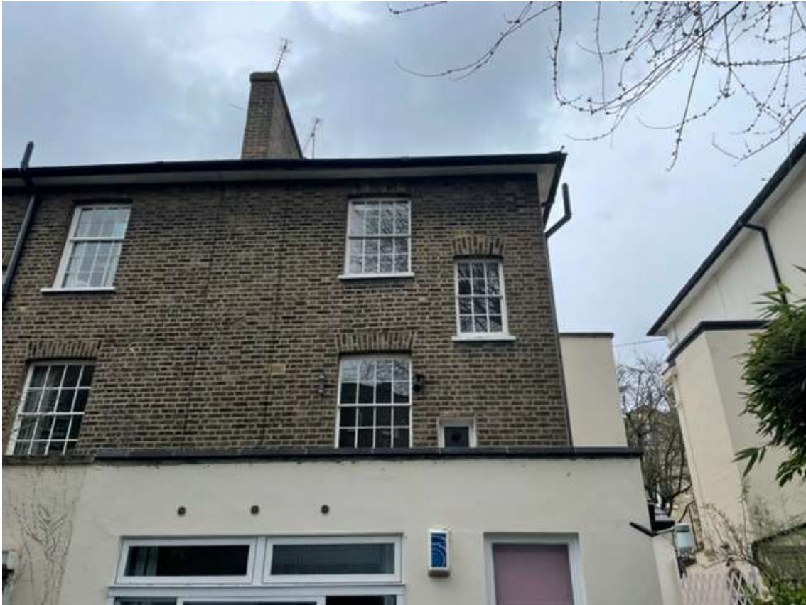
Rear elevation showing lower ground floor extension parapet to 4a
