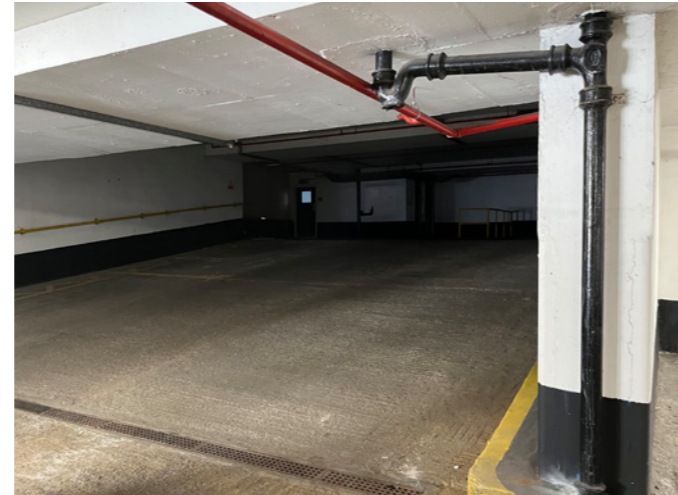
Existing car park ramped slabs
