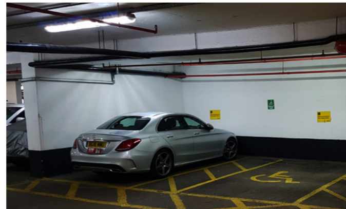
The existing car park relies heavily on artificial lighting
