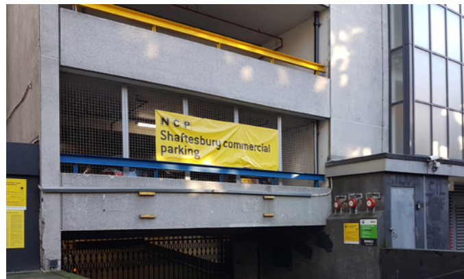
Existing facade opening on the north east corner
