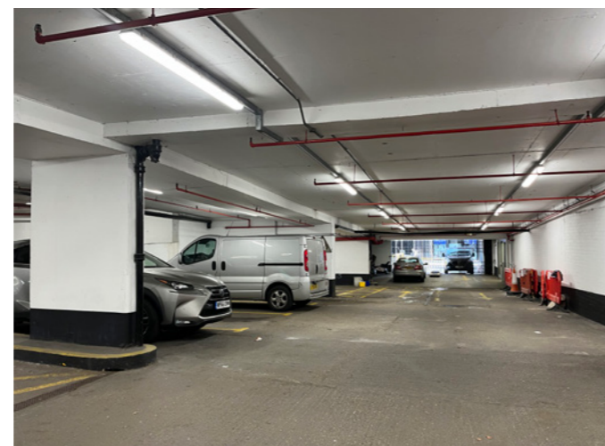
Existing car park deep floorplates
