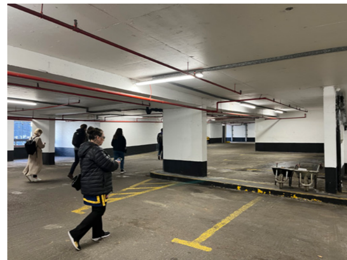
Existing car park restricted floor to ceiling heights
