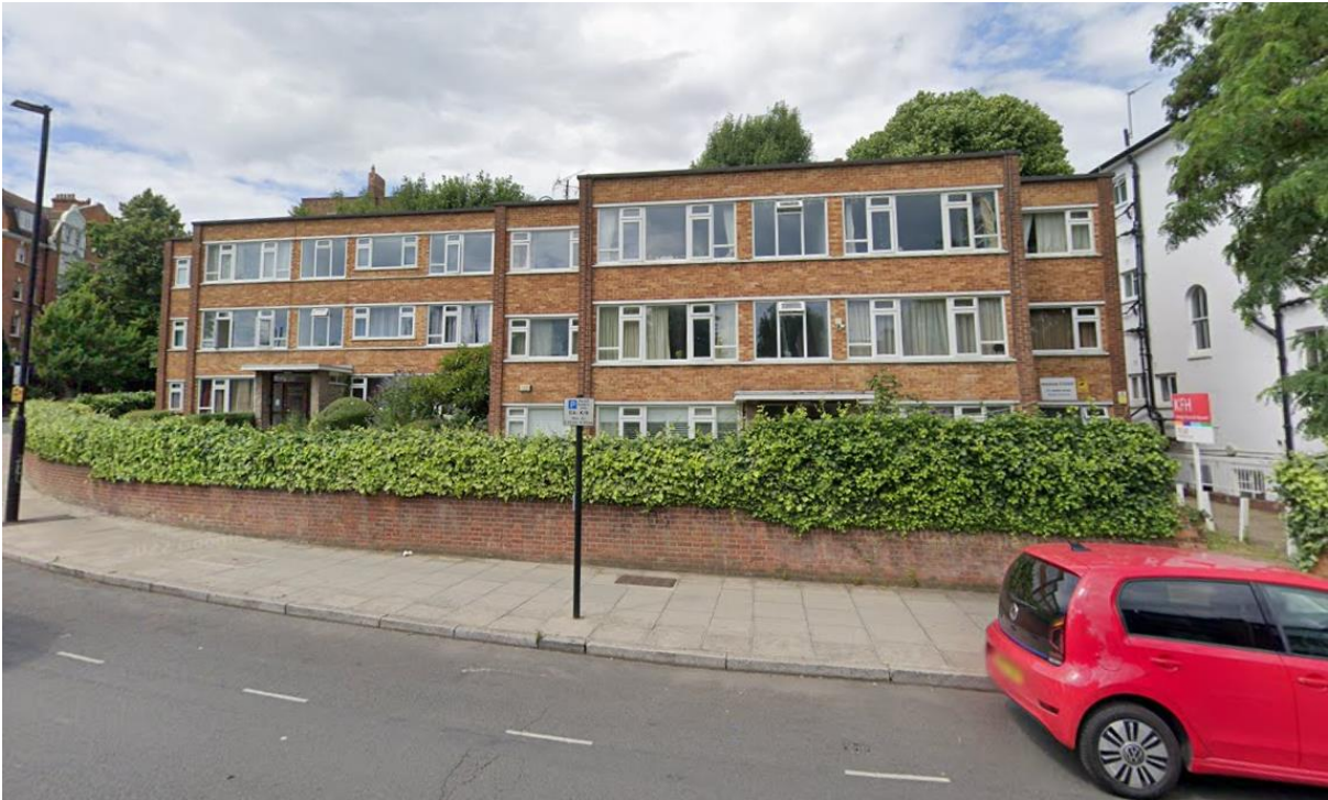
Figure 1: Front elevation of application site (Manor Court). Facing north on Abbey Road.
