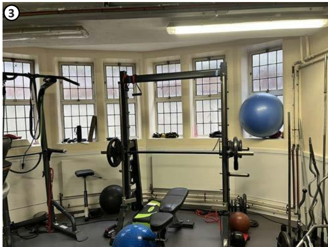
Plate 5 View showing bay window, heating pipes will utilise existing openings shown here on the right.
