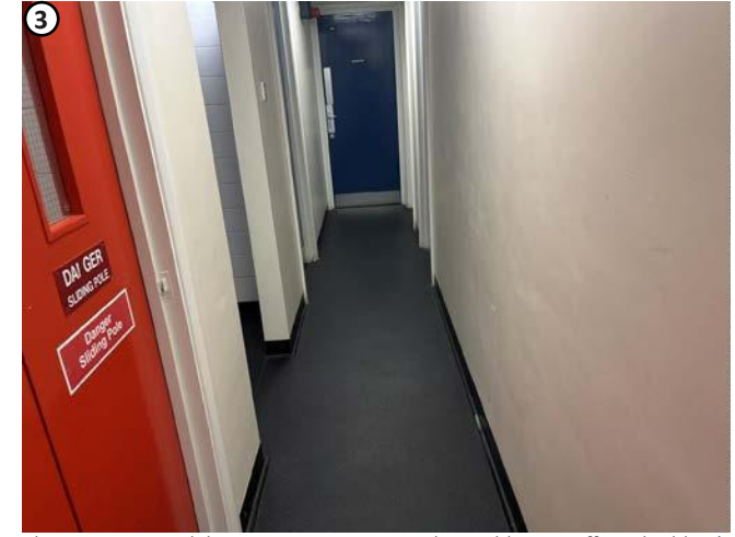
Plate 35 New slab penetration required would not affect building's significance.
