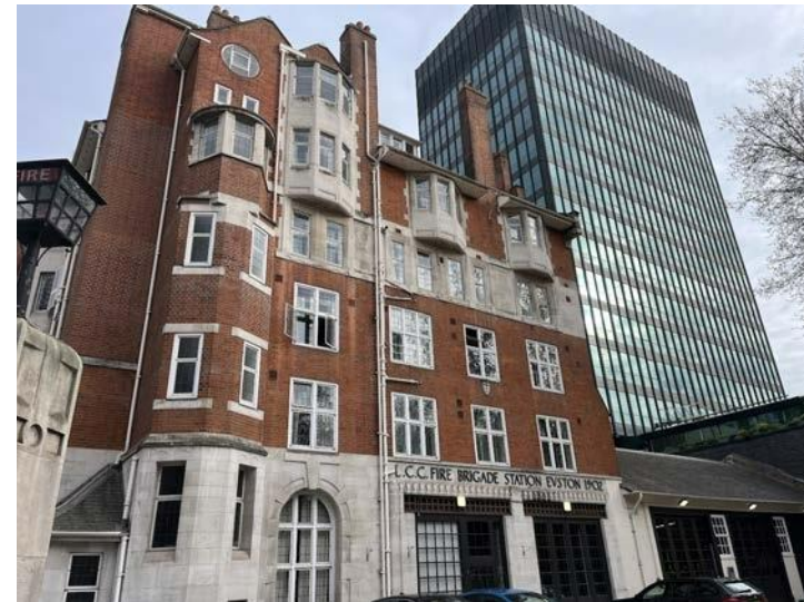
Plate 1 Front facade of the site, as seen from Euston Road.
