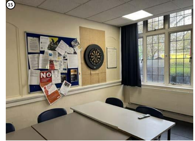
Plate 25 Former yard to stables, now enclosed. Pipe work to radiators to be reused.
