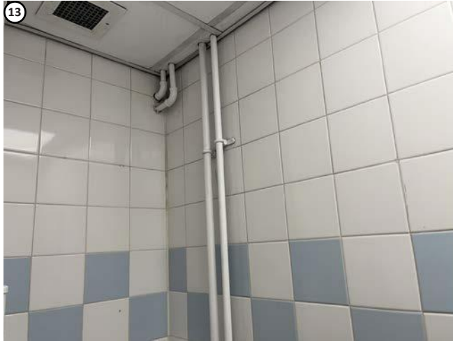
Plate 23 Existing pipe runs to be reused, later fabric of no interest.
