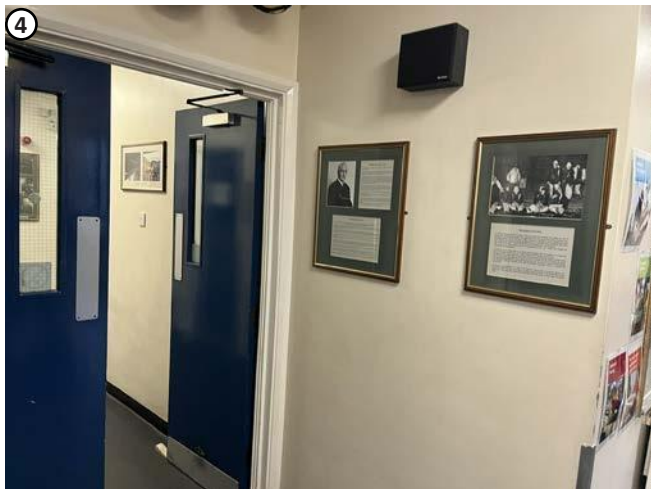
Plate 14 Showing modern fabric installed in previous engine room. High level wall penetration would be hidden in suspended ceiling.
