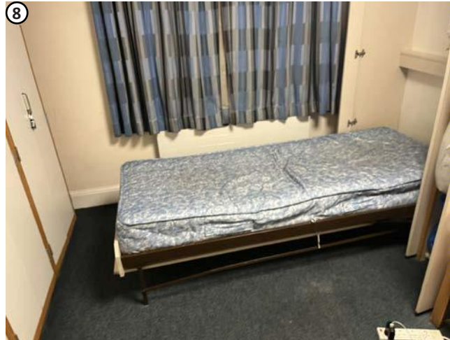
Plate 40 Penetrations for existing pipe work to radiator to be reused where feasible.
