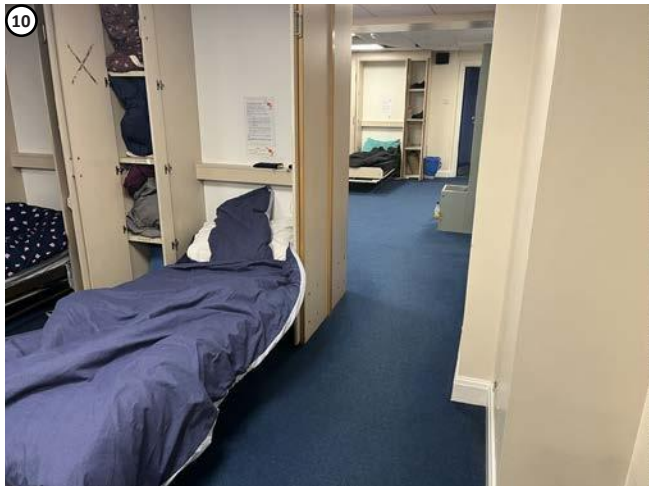
Plate 42 Penetrations for existing pipe work to radiators to be reused where feasible and high level penetration required above suspended ceiling would not affect any fabric of interest.
