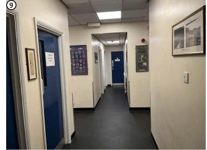
Plate 19 Several high level penetrations required in modern fabric of no interest.
