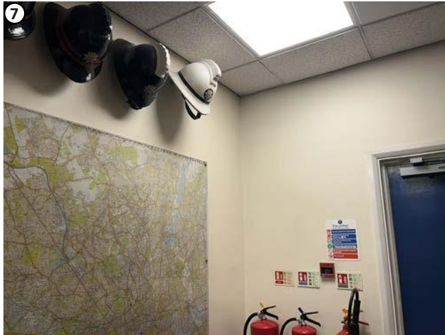
Plate 17 Pipe work above suspended ceilings would utilise existing openings where feasible. Modern fabric visible.
