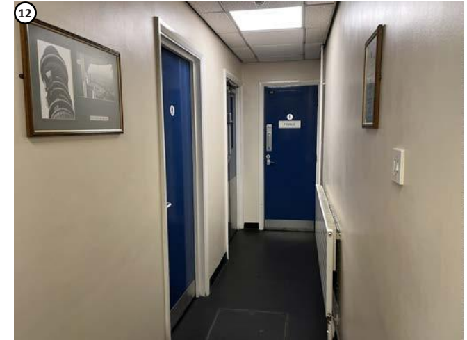
Plate 22 Pipe work to be located above suspended ceiling above far door. Only affecting later fabric.
