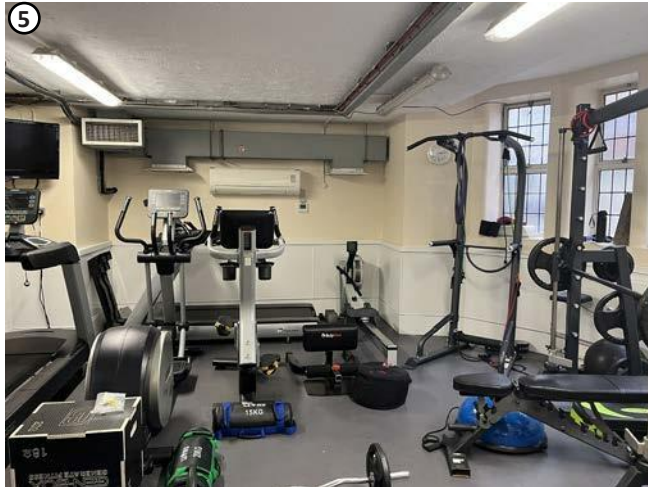
Plate 7 New heating pipes will run to the left of this image utilising existing openings.
