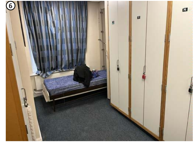
Plate 38 Penetrations for existing pipe work to radiator to be reused where feasible.
