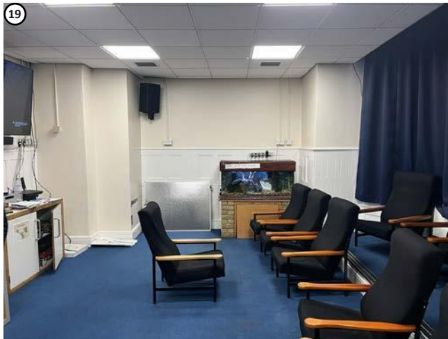
Plate 29 Recreation room showing historic wainscoting. Some slab penetrations required and high level wall opening above suspended ceiling to left. Would not affect any fixtures or fittings of interest.
