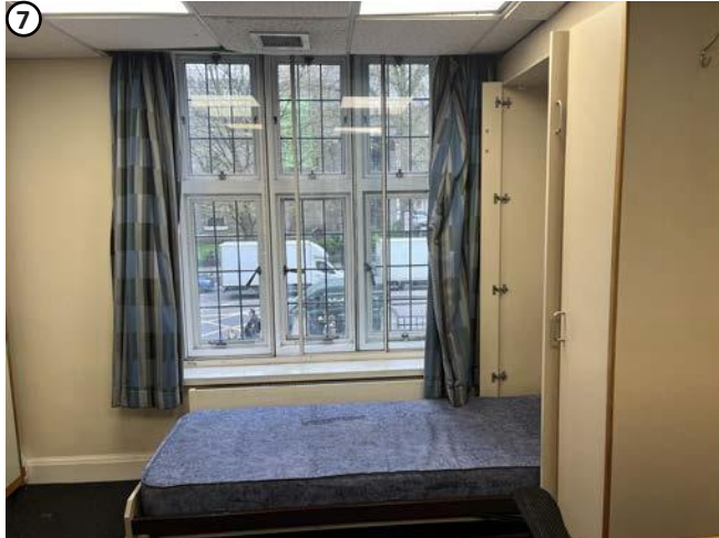
Plate 39 Penetrations for existing pipe work to radiator to be reused where feasible.
