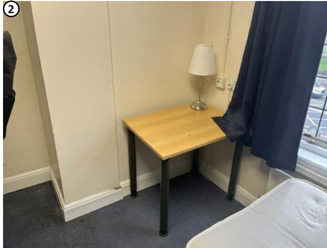
Plate 49 Penetrations for existing pipe work to radiators to be reused where feasible.
