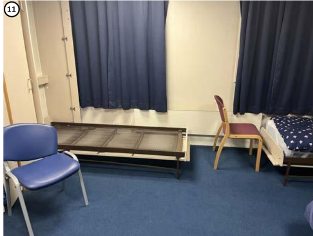
Plate 43 Penetrations for existing pipe work to radiators to be reused where feasible.
