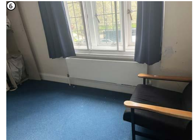
Plate 54 Penetrations for existing pipe work to radiators to be reused where feasible.
