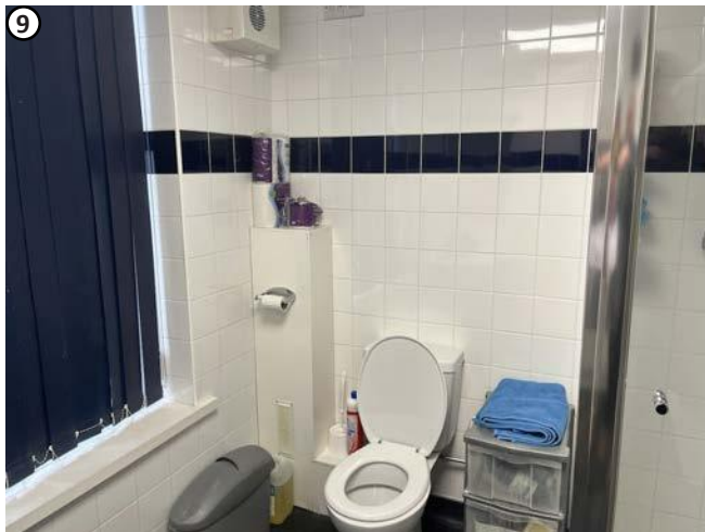
Plate 57 High level penetrations required above suspended ceiling would not affect any fabric of interest.
