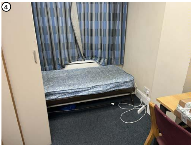
Plate 36 Penetrations for existing pipe work to radiator to be reused where feasible.
