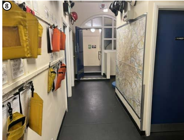
Plate 18 Several high level penetrations required in modern fabric of no interest.
