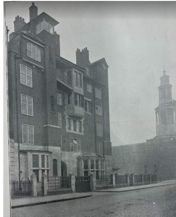
Figure 6 Historic photograph showing Eversholt Street elevation and former carriage arch.
