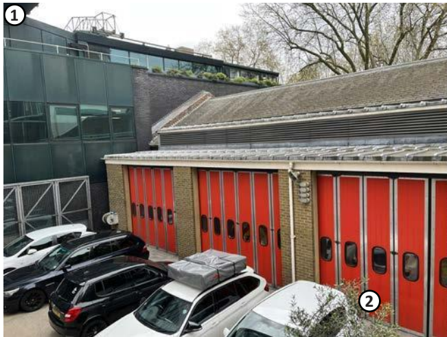
Plate 11 View of 1920s extension. The ASHPs will be located to the left of the image and a penetration made through the bay to the far left, resulting in no negative impact on the significance of the original building.
