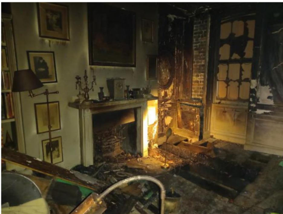
Figure 4.3 This shows the corner which is most fire damaged. The floor and the front wall panelling can be seen to be damaged. The exposed brick face is the part of the wall which did not have panelling before the fire. The fire surround can be seen as fire damaged.
