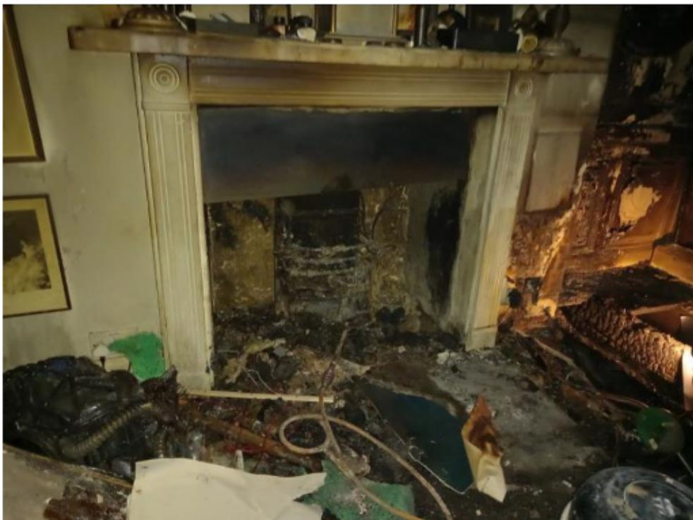
Figure 4.4 Fireplace and surround damage.
