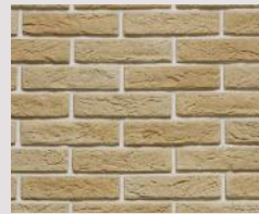
Buff facing brick finish to the sides of new external stair
