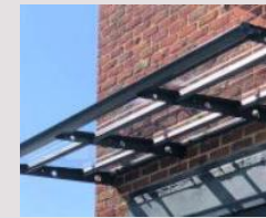
Sheltered entrance with new canopy
