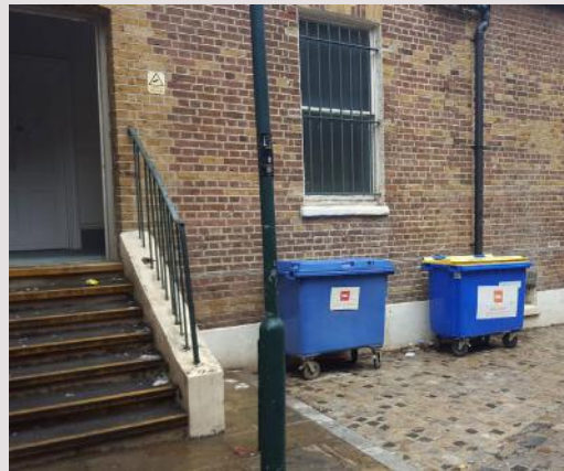
Kerb line stops alongside escape staircase with area for bin storage.
