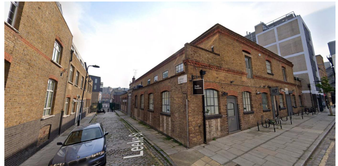
Figure 6 – Street view of 15-17 Leeke Street, Camden, London
