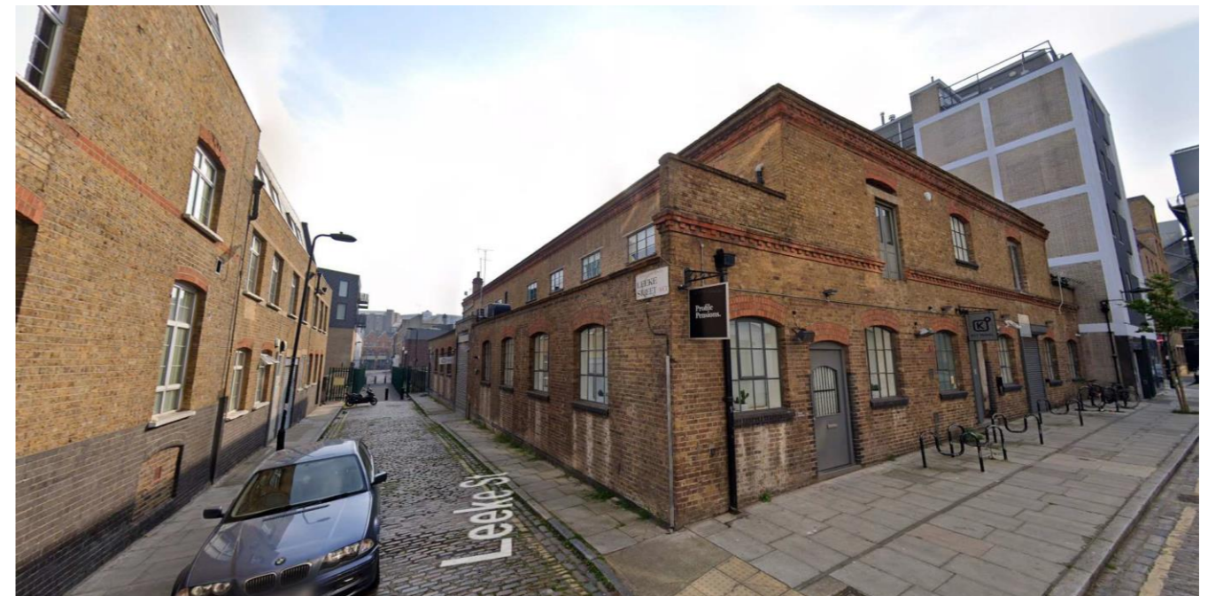
Figure 2 – Street view of 15-17 Leeke Street, Camden, London
