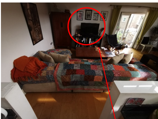
Location of the proposed new window, as viewed from the internal spaces.
