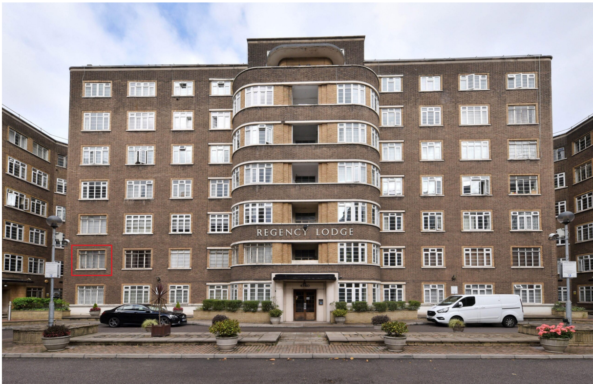
South elevation of the courtyard with the applicant site highlighted in red
