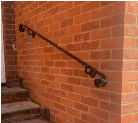
Figure 1 – Black metal railings fixed to masonry
