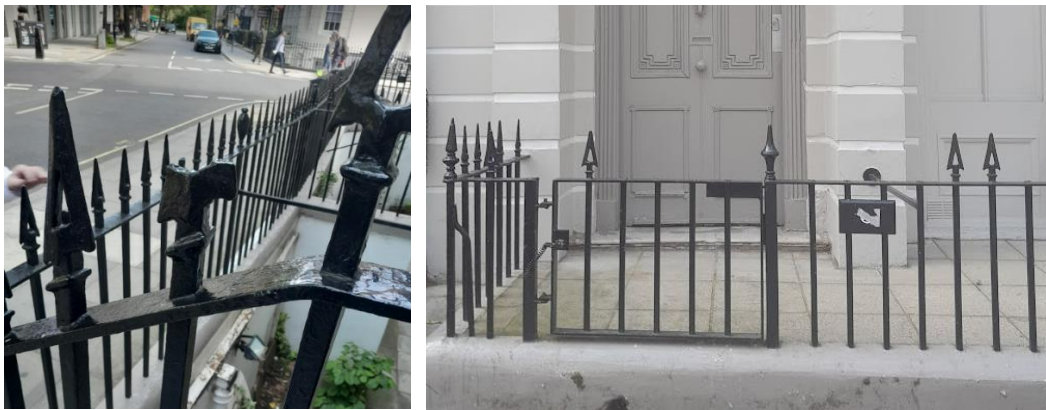
Figure 16. From left: Detail of damaged rail head ; South elevation of The Hotel on Marchmont Street with damaged railings in the foreground.
