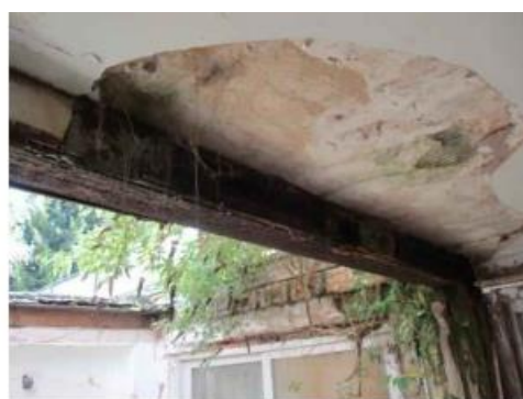
Corroded steel beam
