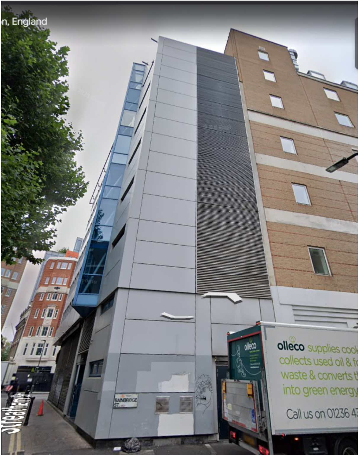
3. Photo of existing Bainbridge Street Elevation
