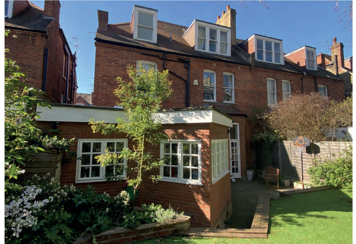
Existing rear view
