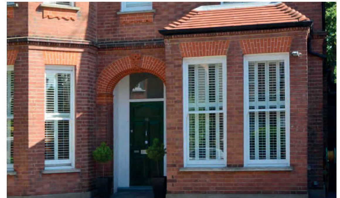
Brick detailing to front of property
