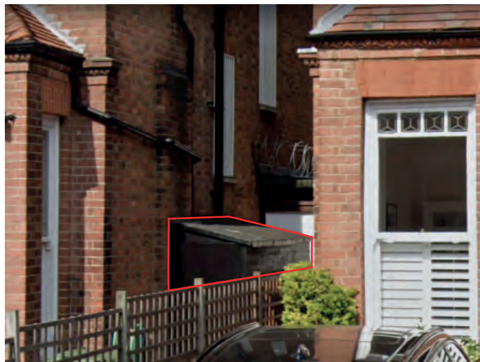
Non-original storage shed to be demolished
