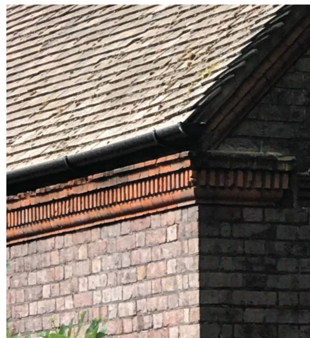
Red brick cornice detail - Existing 38 Frogнал Building
