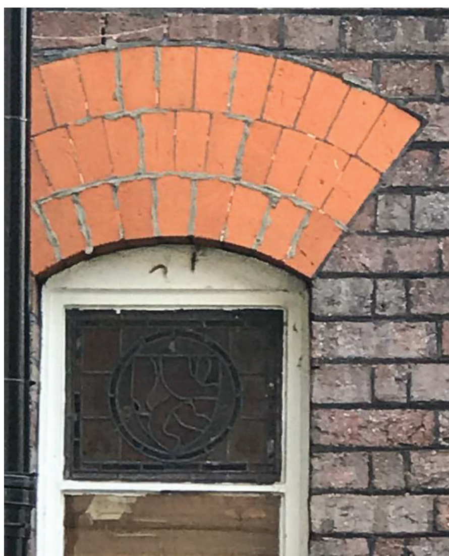
Red brick above windows - 12 Langland Gardens Example
