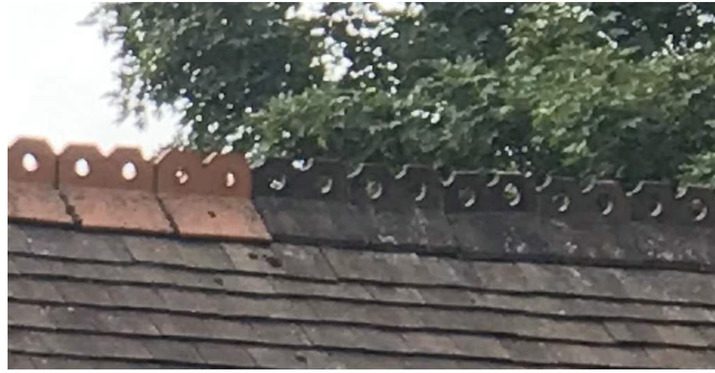
38 Frogнал existing roof ridge tile
