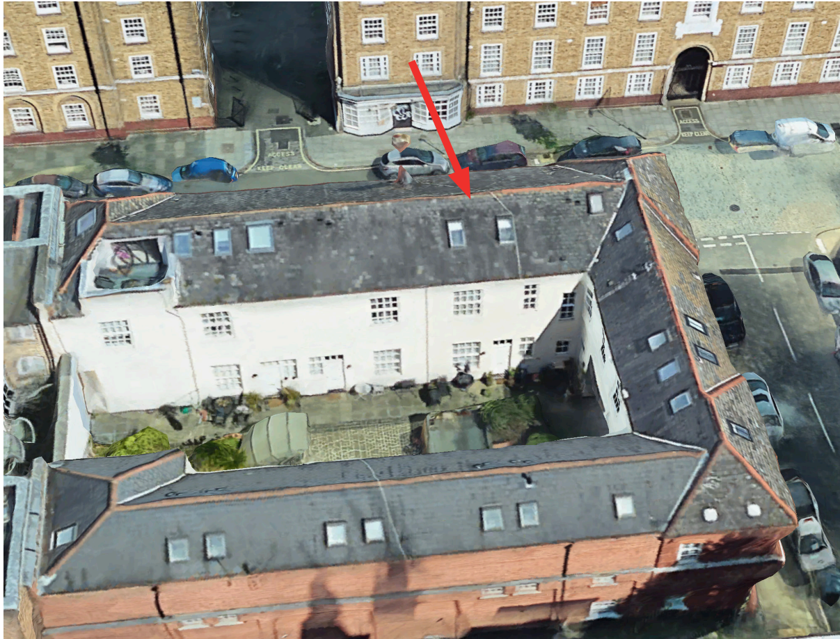
Aerial view of 1-3 Redhill Street Source: Google Earth
