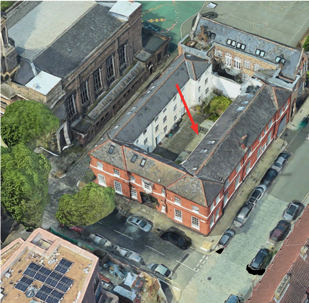
Aerial view of 1-3 Redhill Street Source: Google Earth
