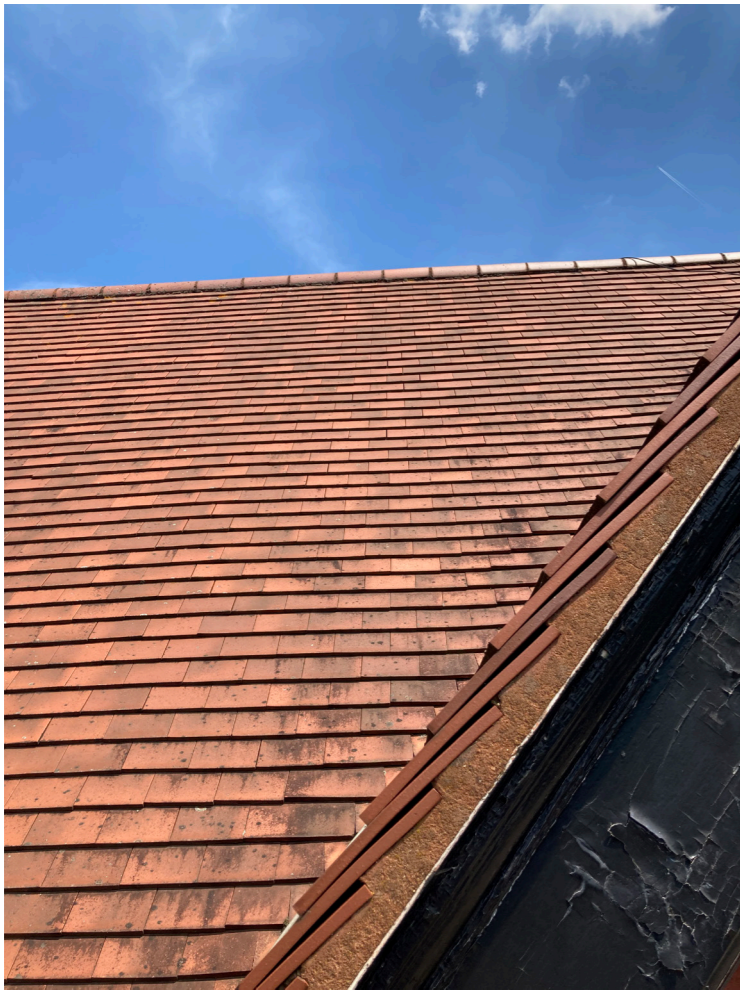
Image of Existing Red Clay Tiles to Roof
