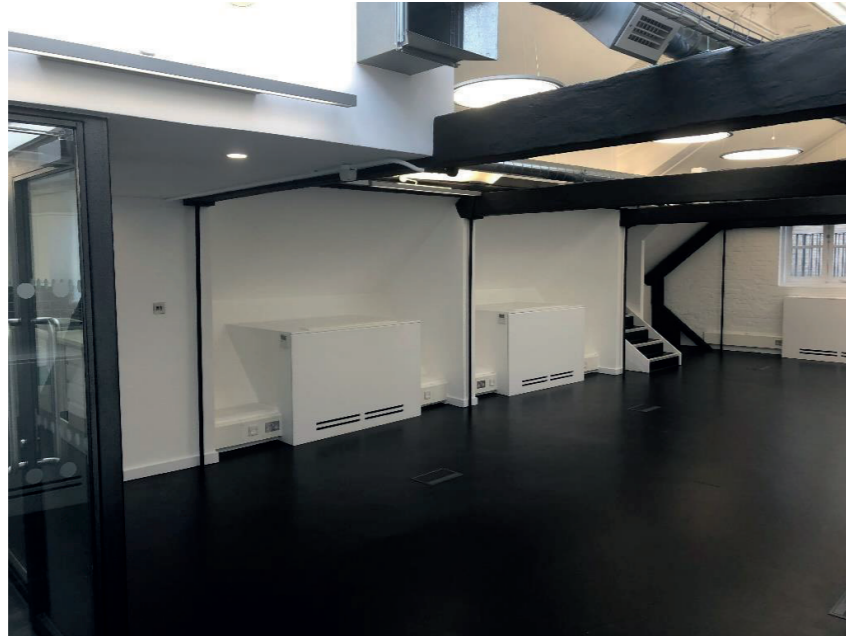
Figure 3.7: Exposed historic timber framing at third floor level
