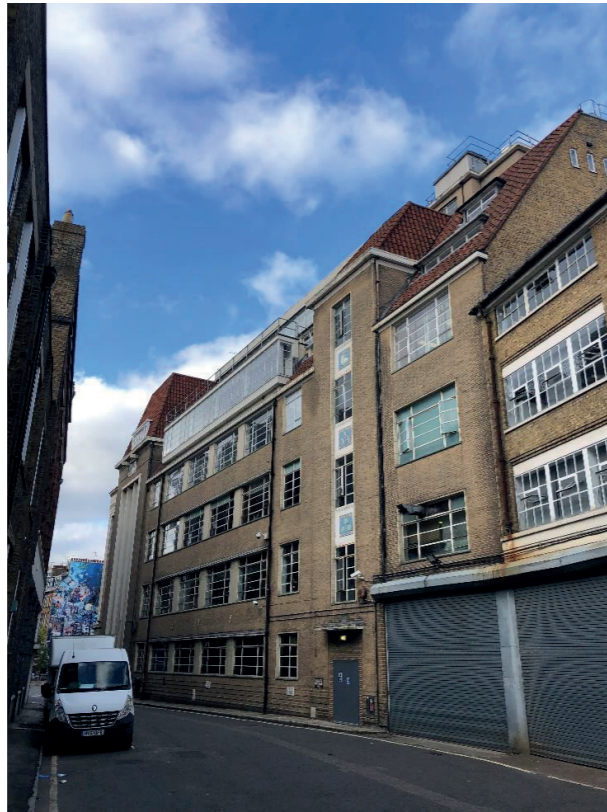
Figure 3.24: View of the Site as found today (south elevation along Alfred Mews) – secondary elevation)
