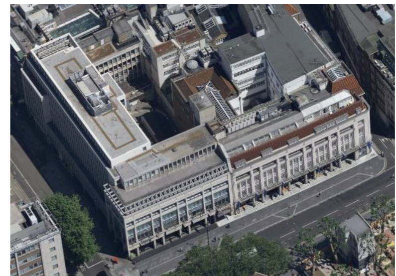
Figure 3.12: Birds Eye View looking east shows principal elevation along Tottenham Court Road and Torrington Place
