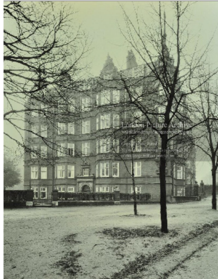
Archive photograph of The Pryors Block A (view from West)
