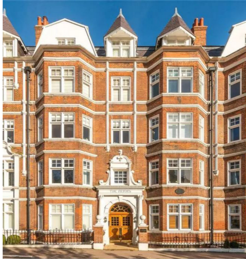
Front Entrance /Elevation Block A
