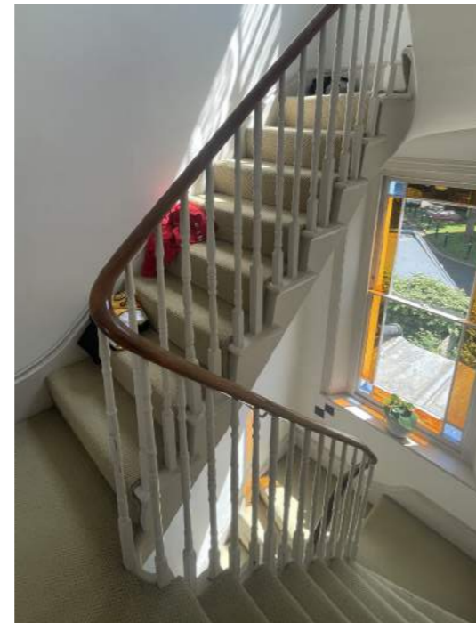
6) EXISTING STAIRCASE TO BE REPLICATED
