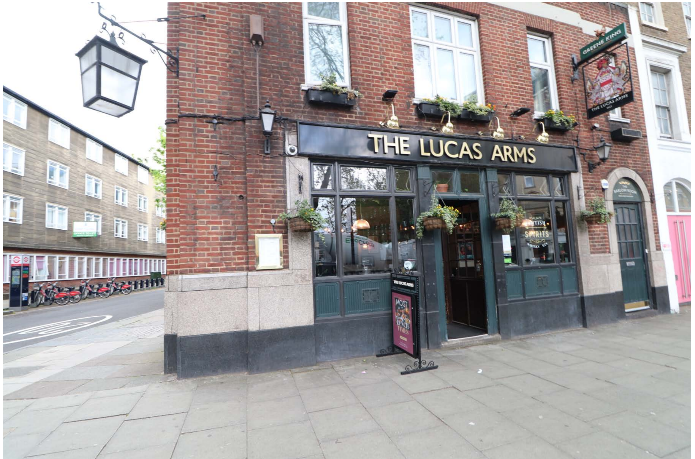
Front Elevation existing photo
