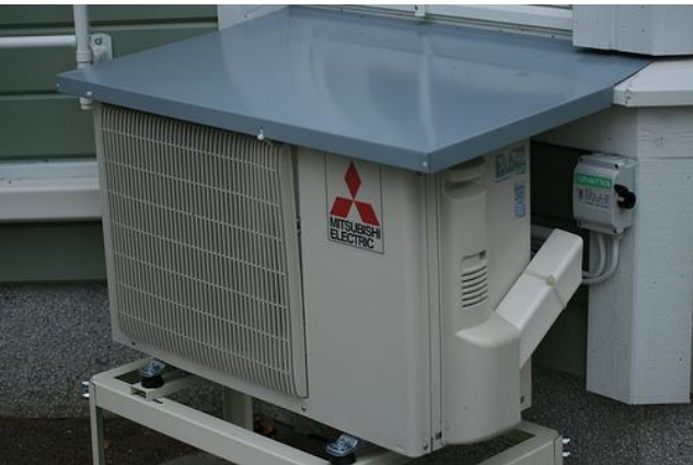
Figure 3: Outdoor unit of an ASHP
