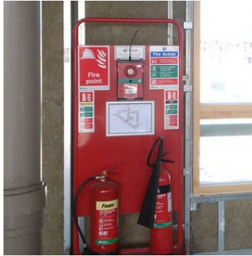
Wireless fire alarm system
