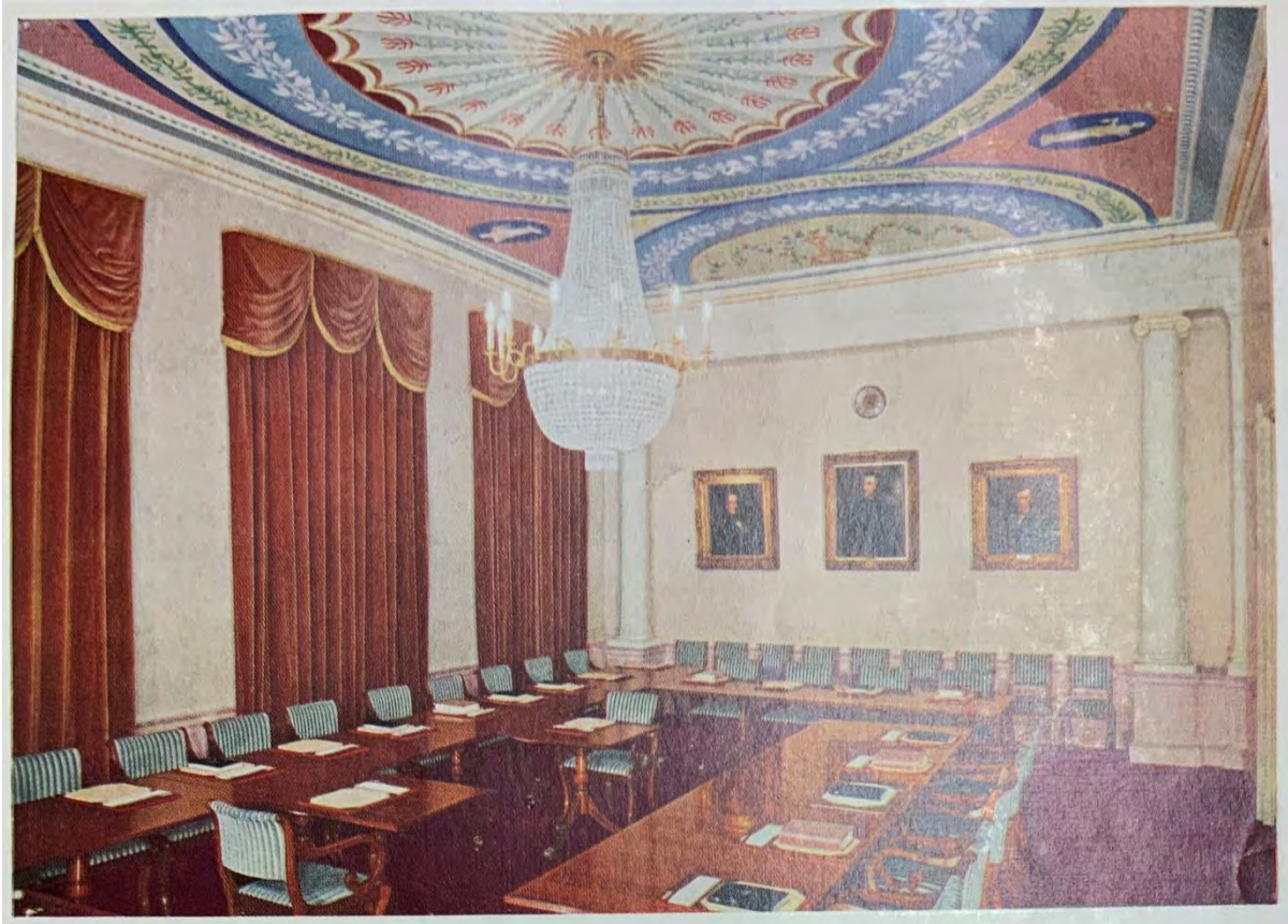
Figure 20: First floor front room with the 18 th C painted plaster ceiling. Note the chimney breast from the rear wall was removed in the mid-20 th C and replaced with the two ionic pilasters and entablature (concealing structural interventions). (Source: Camden Archives).
