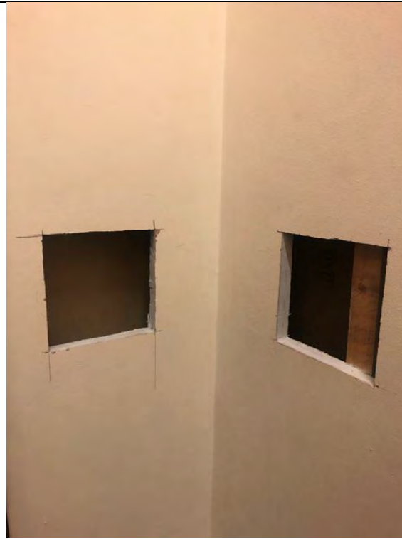
Figure 40: Two small opening up works on wall dividing the former ground floor octagonal room – these works show this is a lightweight modern timber/ plasterboard partition.
