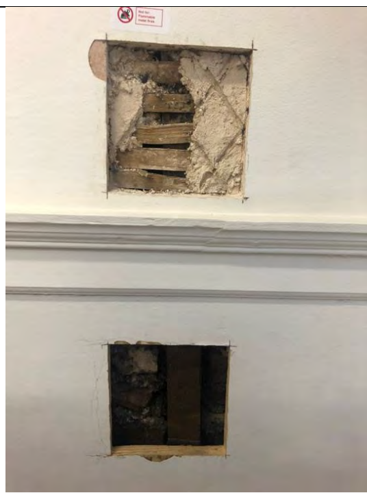
Figure 35: Opening up works undertaken in the existing reception area above and below the dado rail. Above the dado rail there is lath and plaster and below the dado rail, exposed stud with brick either side.
