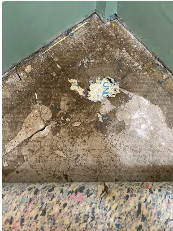
Figure 48: Temporary pulling back of carpet and lining revealed carpet underlay (glue and screed) with the original Portland stone finish below.
