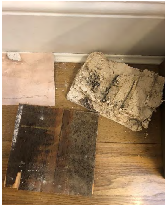
Figure 37: Picture of the cut out pieces showing the plaster from the opening up works above the dado rail and timber board below.
