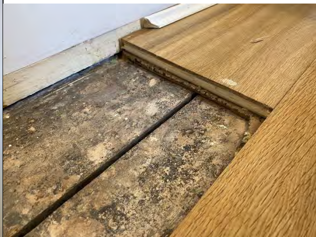
Figure 39: Close up view of the modern board laid on top of early floorboards.
