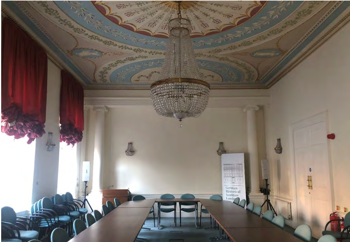
Figure 24: Conference room at first floor. This room retains the 18 th C plaster ceiling and doors from the 19 th C remodelling. The Ionic columns and entablature dates from the mid-20 th C refurbishment when the chimney breast was removed.
