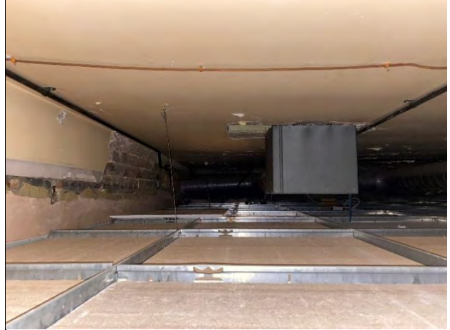
Figure 44: View of ceiling structure and void. Note the concrete slab from the mid-20 th C which replaced the 19 th C timber roof structure here.
