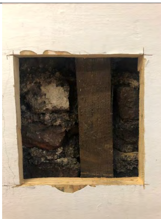
Figure 36: Closer view of opening up works in reception area wall below the dado rail showing the stud and exposed brick. Below the dado rail is a timber board rather than plaster.
