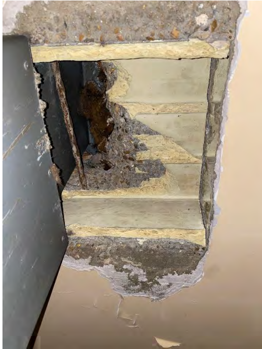
Figure 43: Small existing opening reveals the concrete slab in this area.
