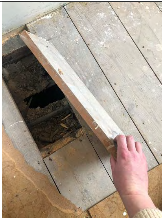
Figure 46: Depth and profile of the timber boards in first floor conference room.
