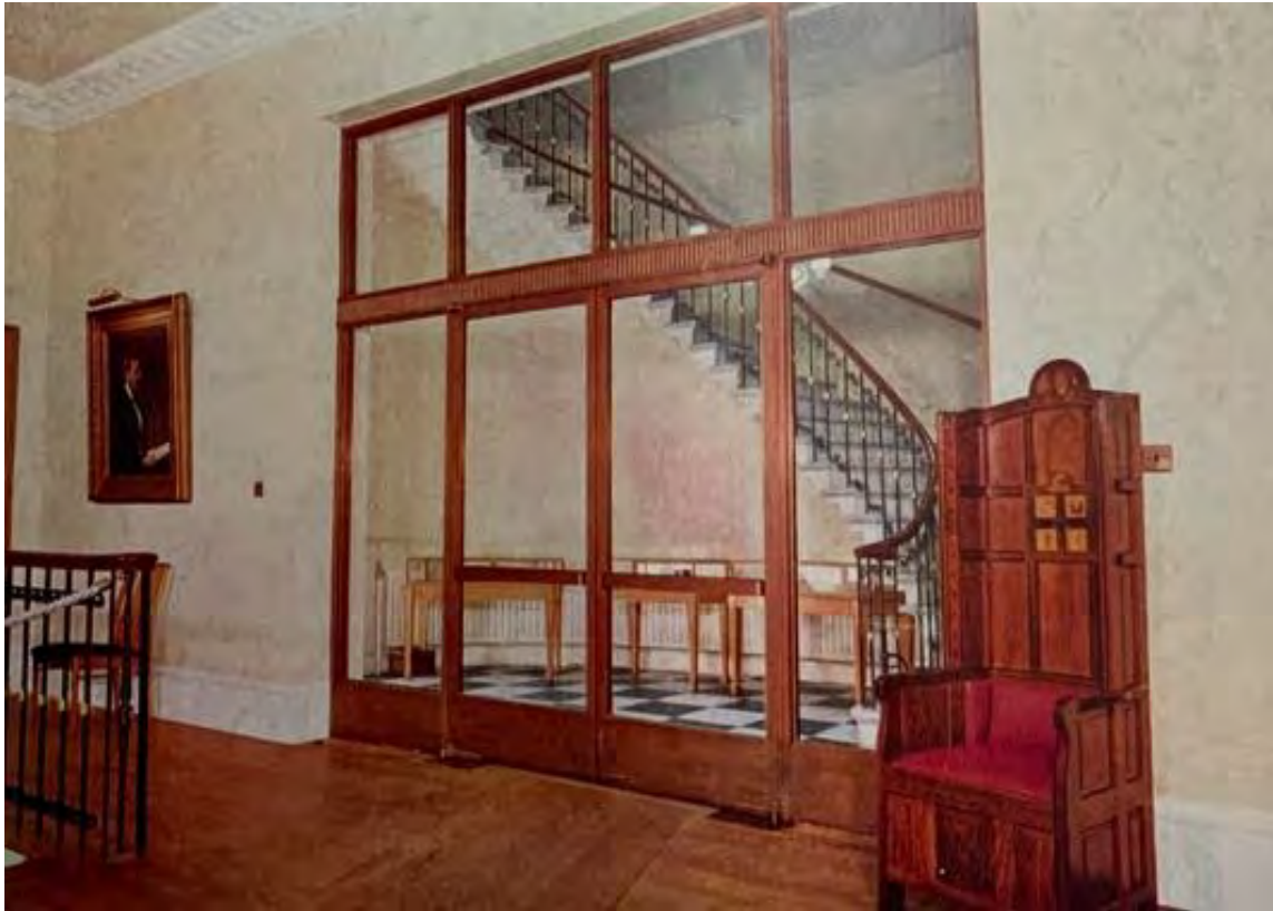
Figure 18: Ground Floor rear room, showing the large, glazed opening between this room and the stairwell. This opening dates from the mid-20 th C and was infilled during the c.1990s works (Source: Camden Archives).
