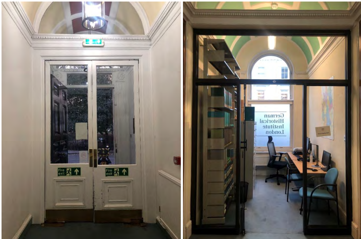
Figure 22: The existing principal entrance from Bloomsbury Square (left) and the 18 th C entrance from Great Russel Street (right). The latter entrance was blocked up in the 19 th C; and moved further west along the façade.
