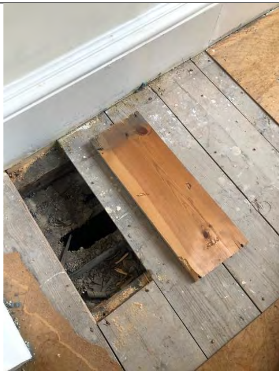
Figure 45: Temporary lifting of carpet and lining in first floor conference room revealed relatively modern pine floorboards.
