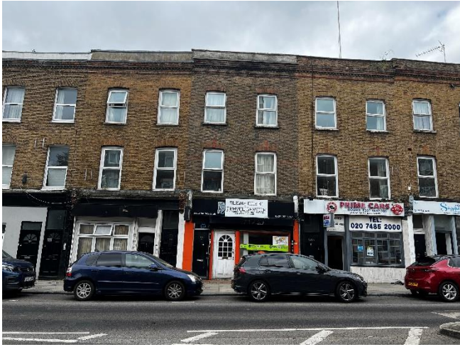
S facing view of the site's frontage
