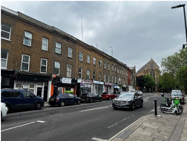
W facing view along Malden Road
