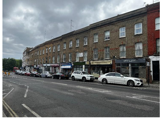
SE facing view of the neighbouring properties
