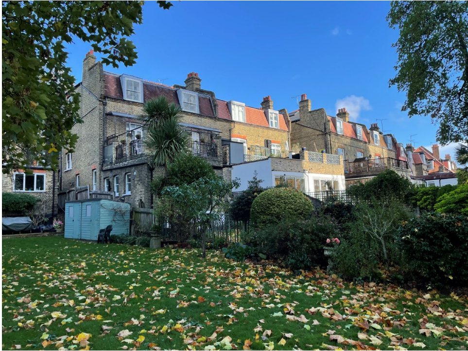
View of the rear / side boundary and of other first floor terraced areas along the terrace
