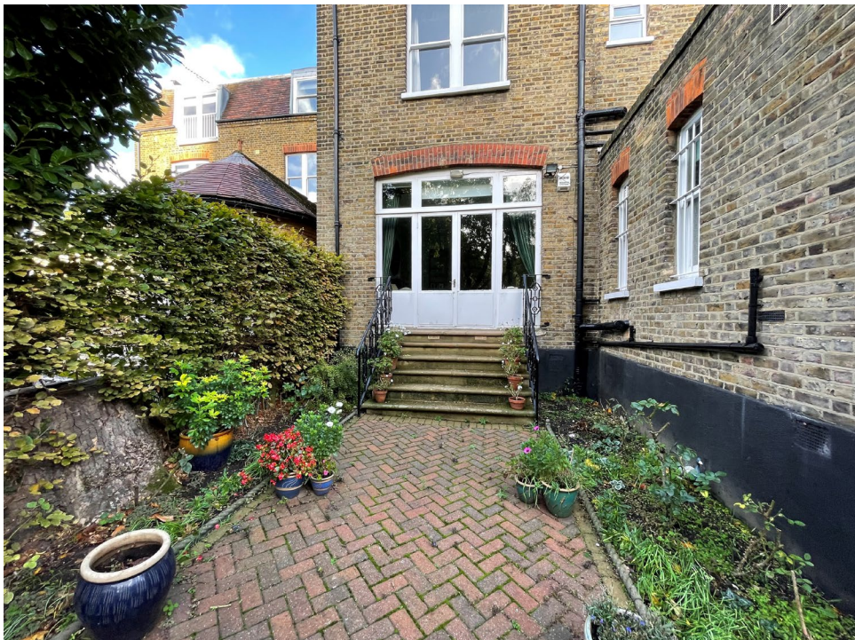
View of the rear / side boundary
