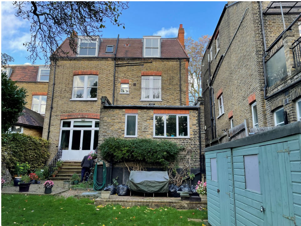
View of the rear elevation and of the existing flat roof
