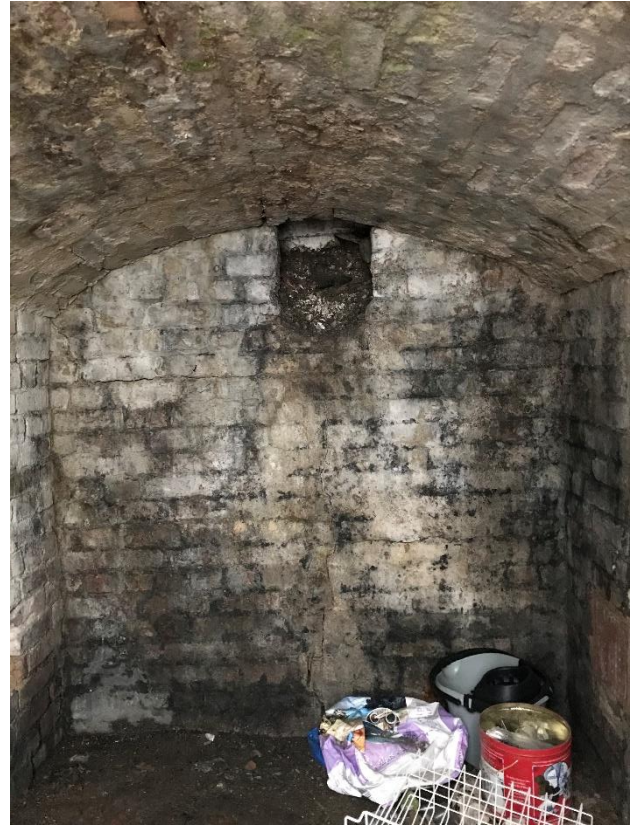
Interior of one of the vaults, with coal shute on the rear wall
