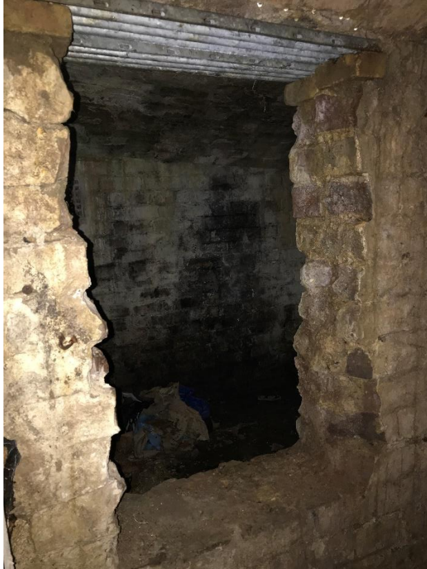
Hole in wall of vault leading to internal of property
