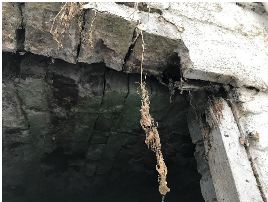
Retaining wall separated from vault ceiling
