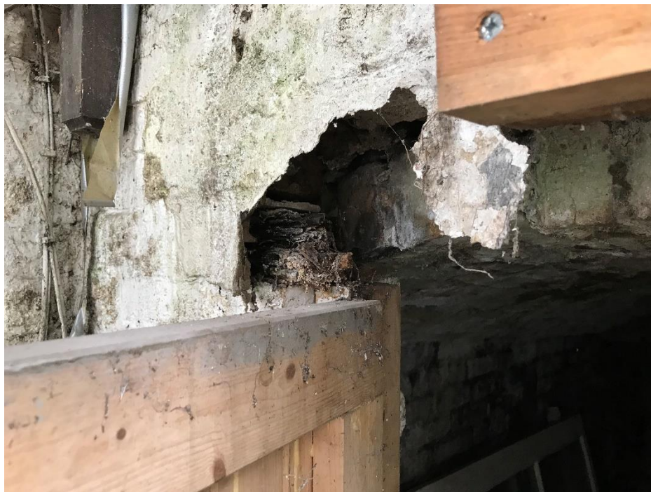
Cavity left following original lintel rotting away
