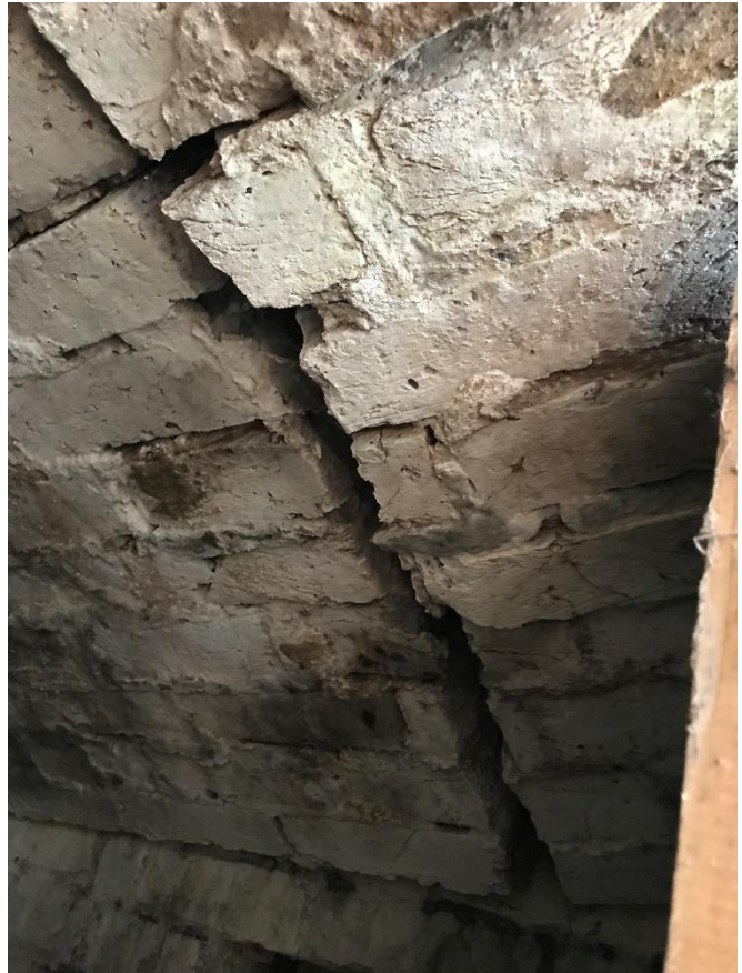
Severe cracks in the existing arches
